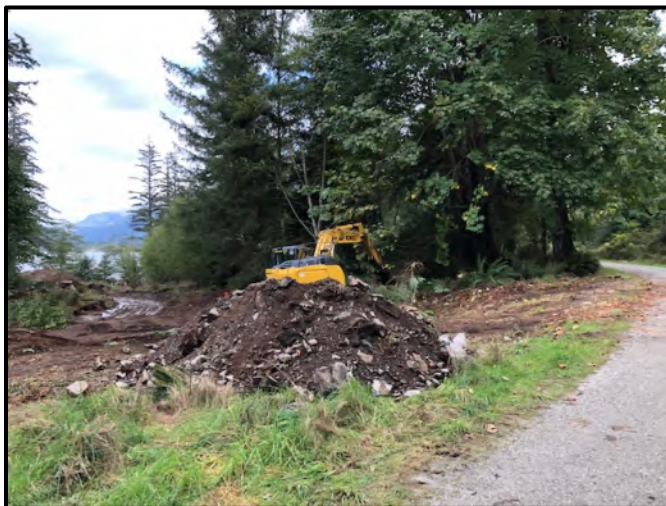
Views of new access lane leading into subject property
