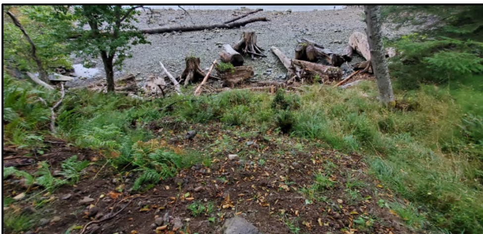
View looking north down steep 6-7m high embankment to the foreshore below.
