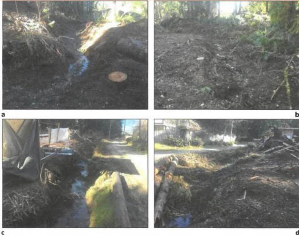
Figure 3, view of Ditch 1 downstream of the Pond outlet (a) and upstream from the junction with Ditch 2 (b). Ditch 2 downstream from the top of the ditch (c) and upstream from the junction of Ditch 1 (d). There was minimal water in both ditches at the time of the assessment.
