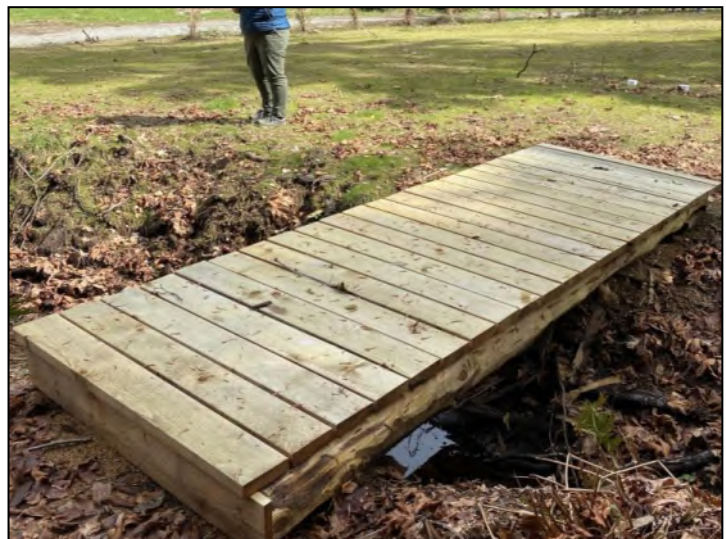
Right: Bridge across ditch.
