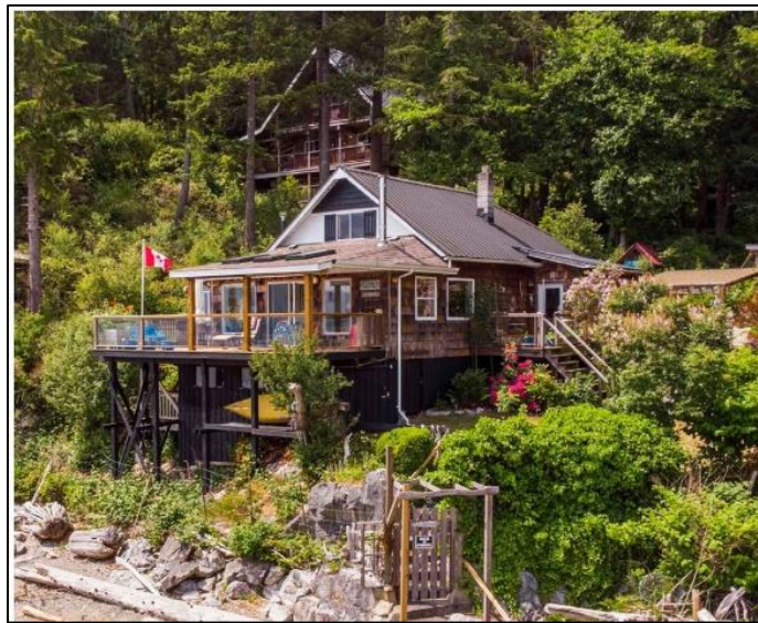
Figure 1 - View from foreshore, secondary dwelling background
