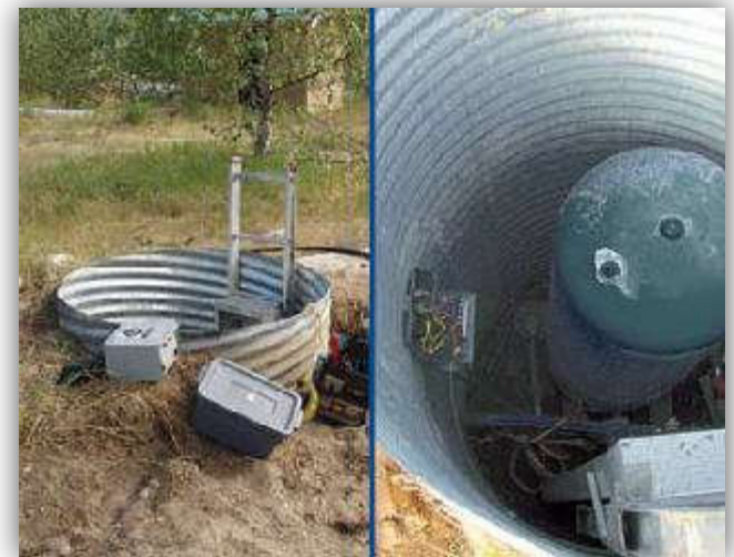
DrilledWells in Pits
