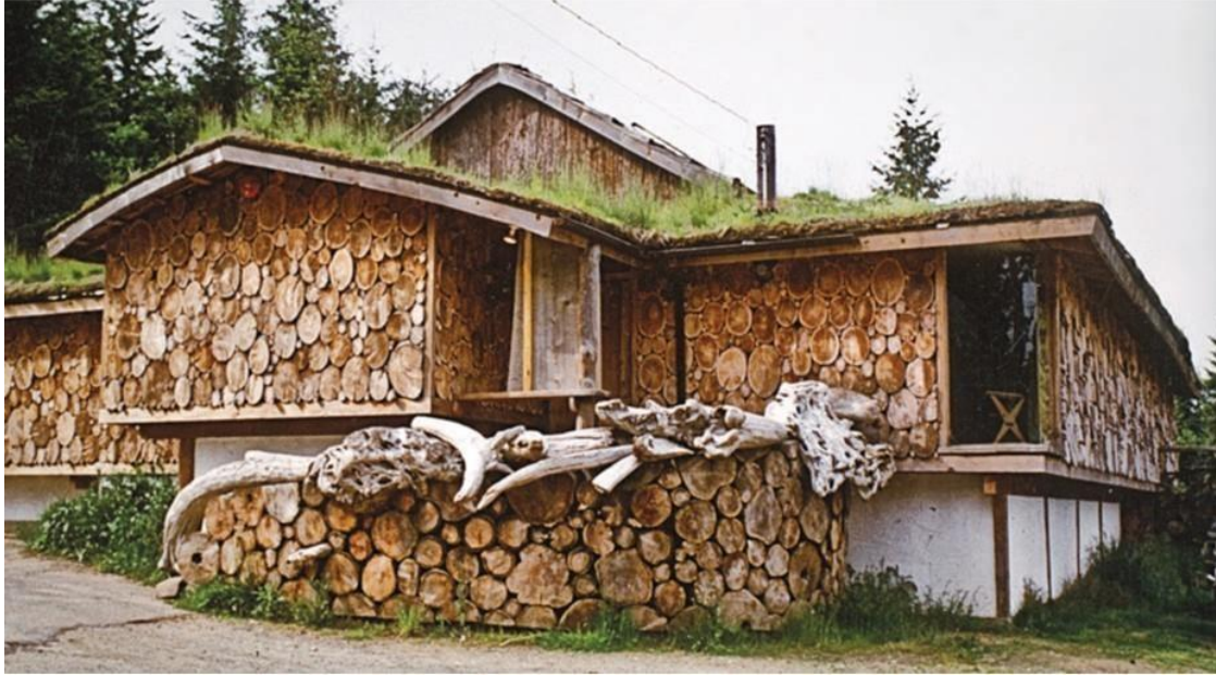
Figure 6. Close up view of the log-round exterior siding on the Green Roof addition. Source: Kahn 2008: 34.
