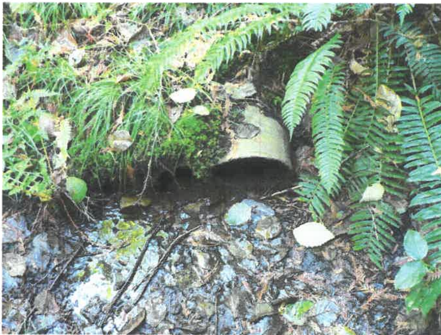
Photograph 8. View of culvert inlet under old road on the east side of property.
