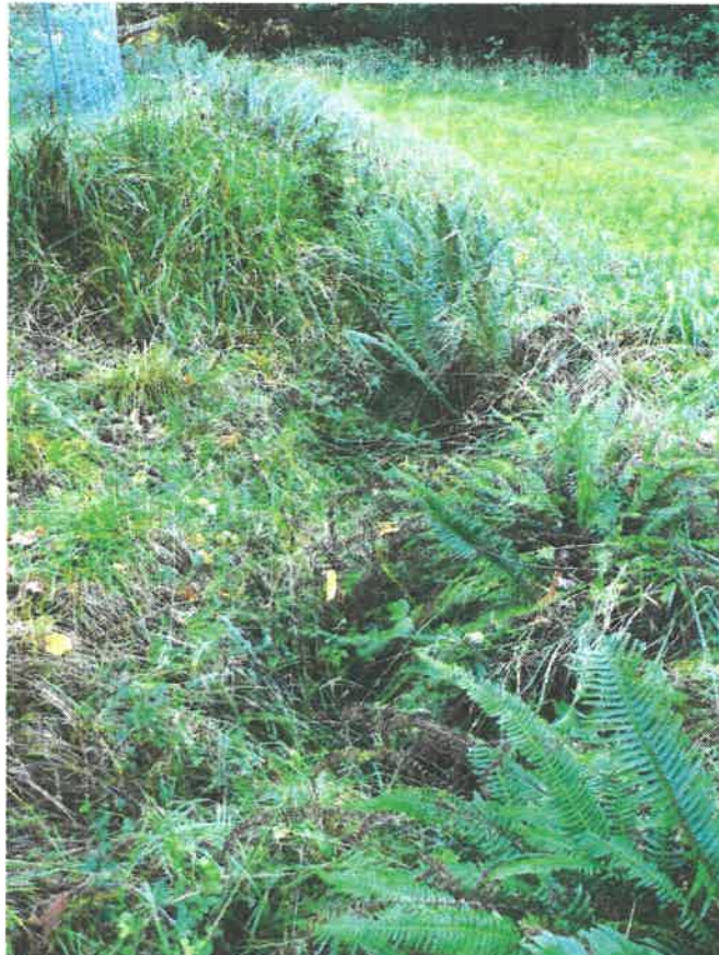
Photograph 1. View of poorly defined, vegetated ditch flowing west to east across 4330 Central Road.
