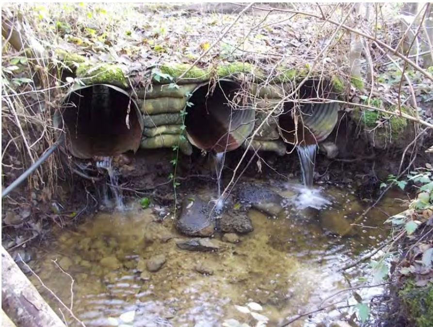
Looking upstream at the culverts that direct the stream under a residential access road.
