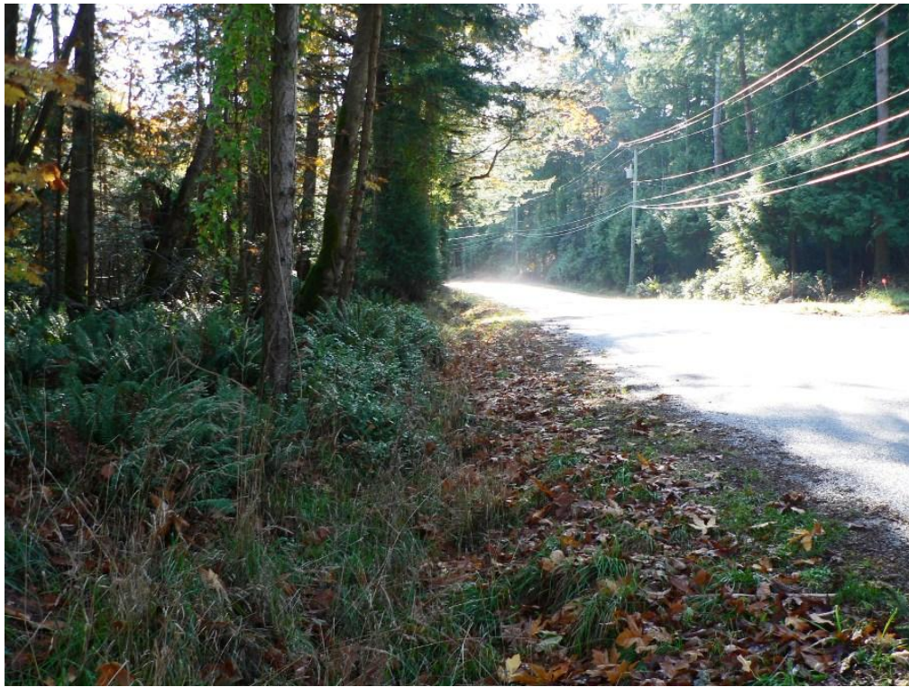
Photograph 7. View downstream on poorly defined ditch / swale along Central Road.
