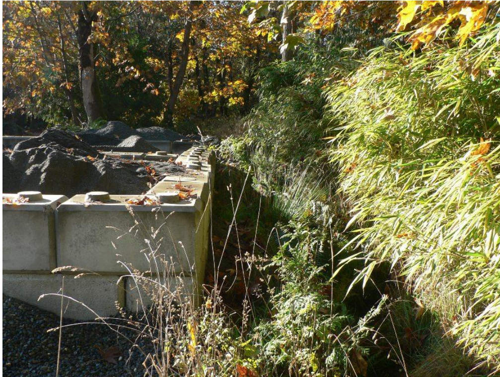
Photograph 3. View downstream along the rear of the bulk storage bays with ditch on right.
