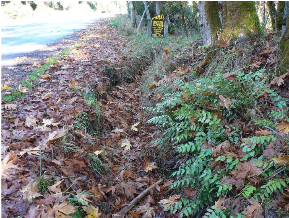
Photograph 6. View upstream from Central Road to where ditch enters from subject property.
