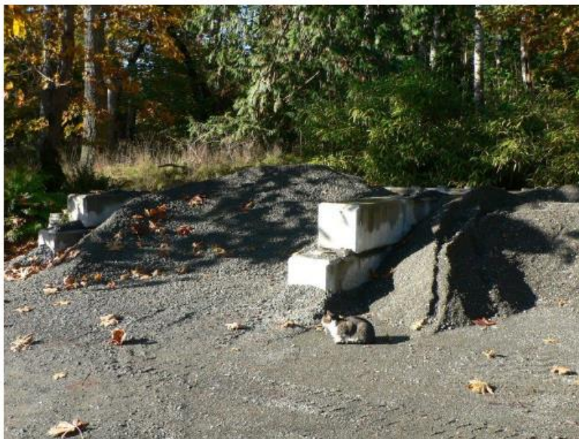
Photograph 2. View of concrete lock-block containment with gravel.
