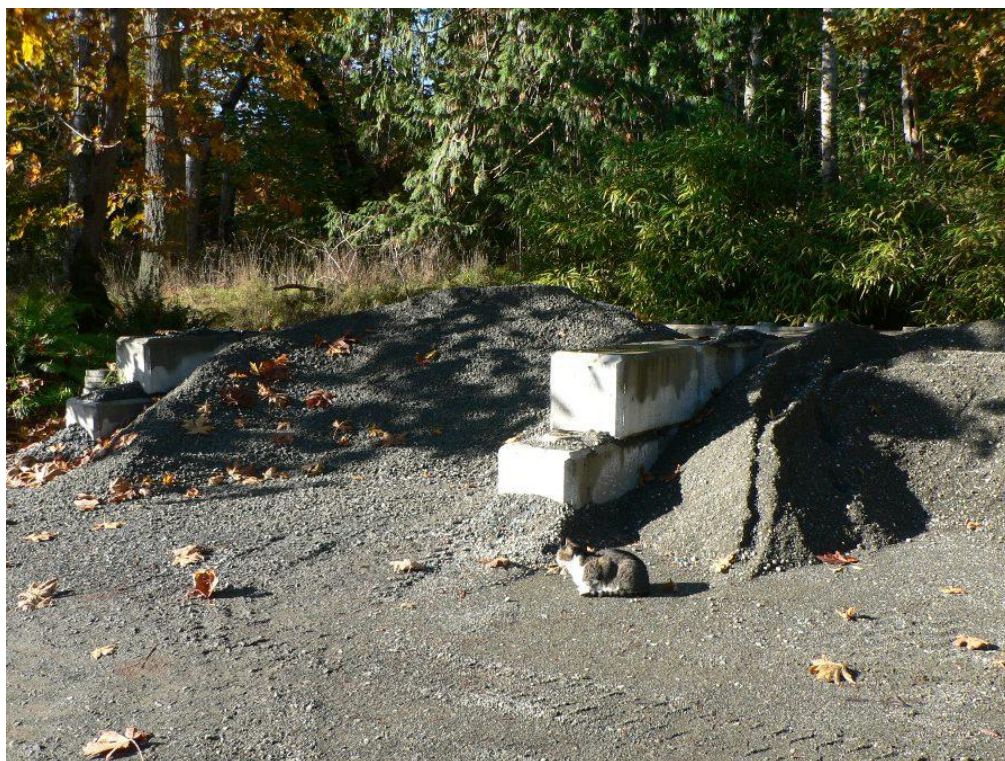
Photograph 2. View of concrete lock-block containment with gravel.
