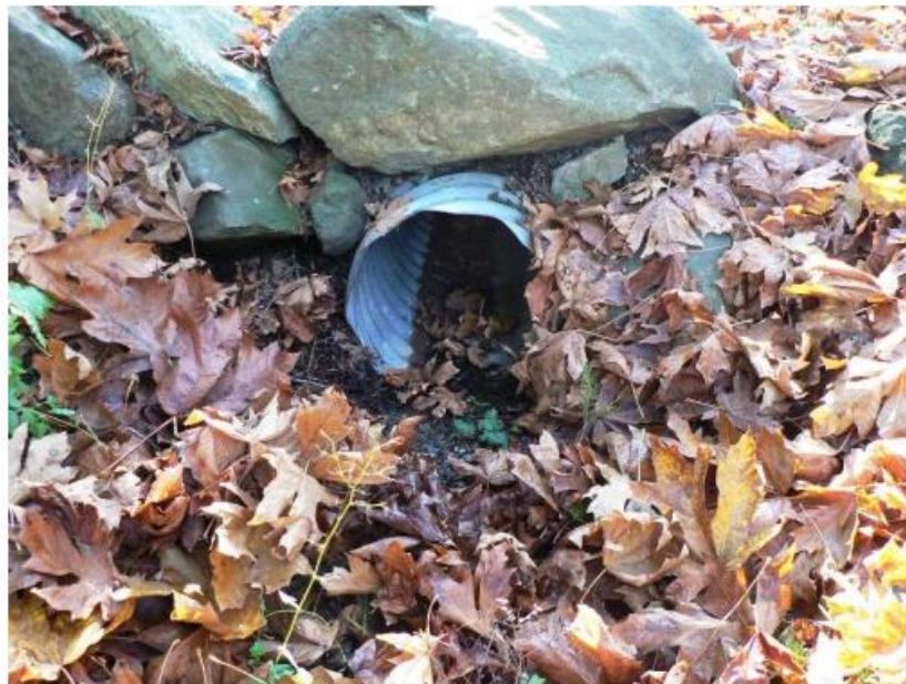
Photograph 8. View of staining on driveway culvert indicating typical water level.
