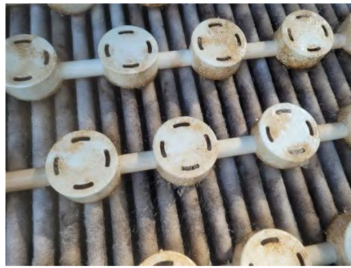
AX20 – orifice shield distribution
