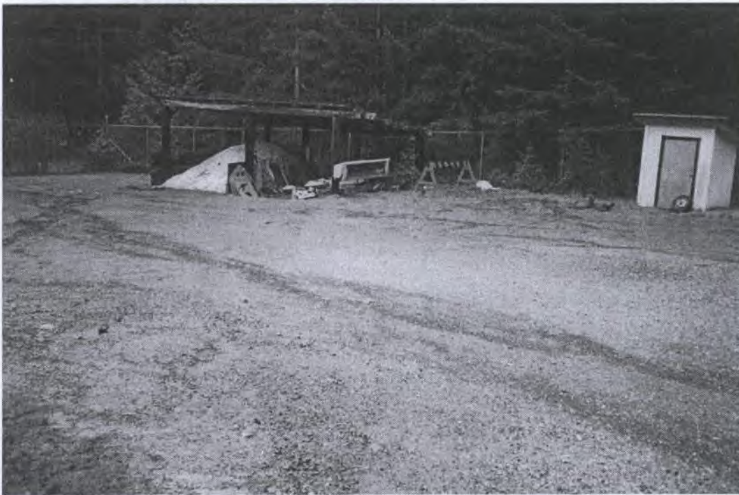
Photo 1: View of pumphouse and highways yard showing salt storage shed.
