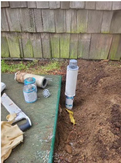
AX20 – carbon filter vent replaced
