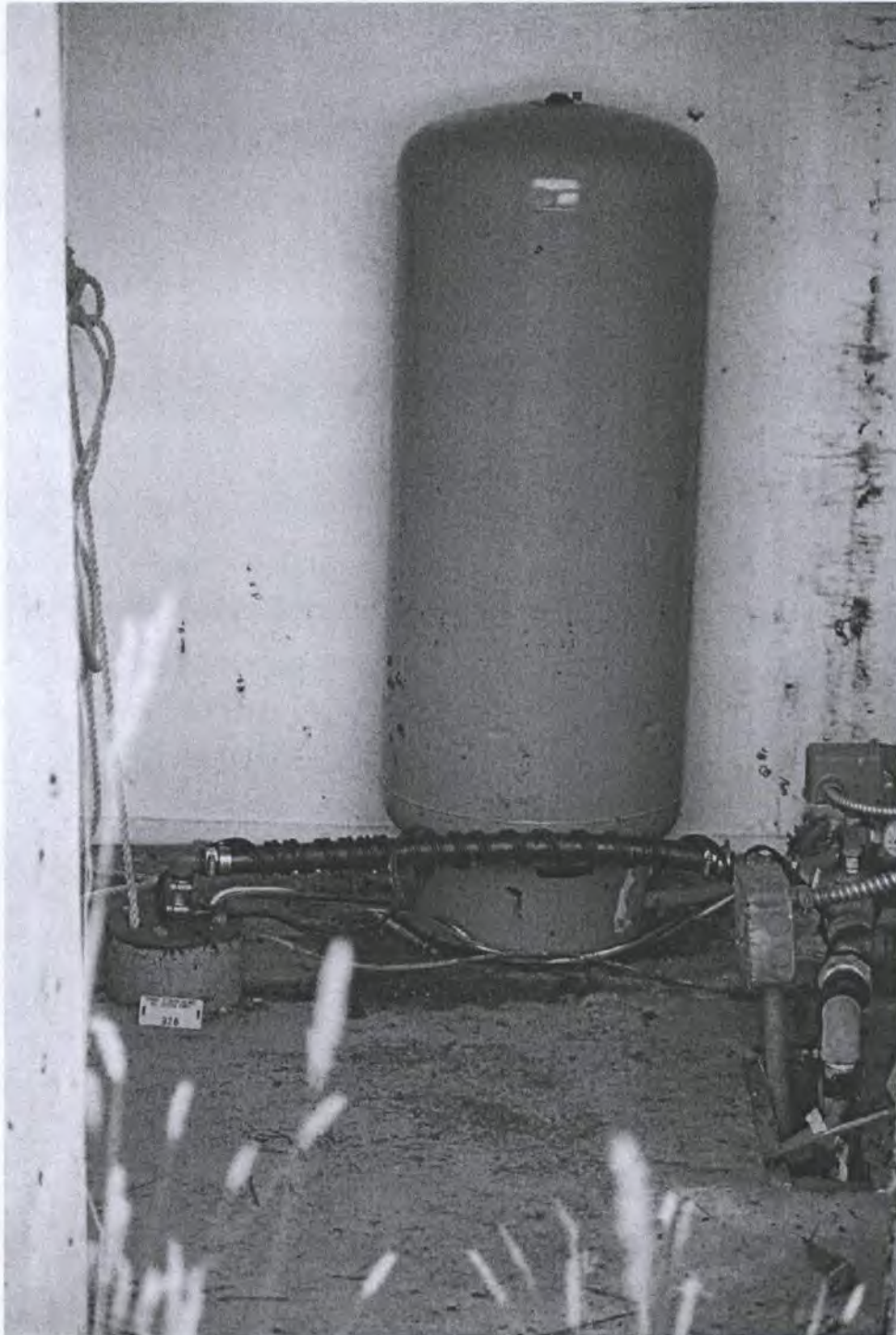
Photo 3: Well and pumphouse interior.
