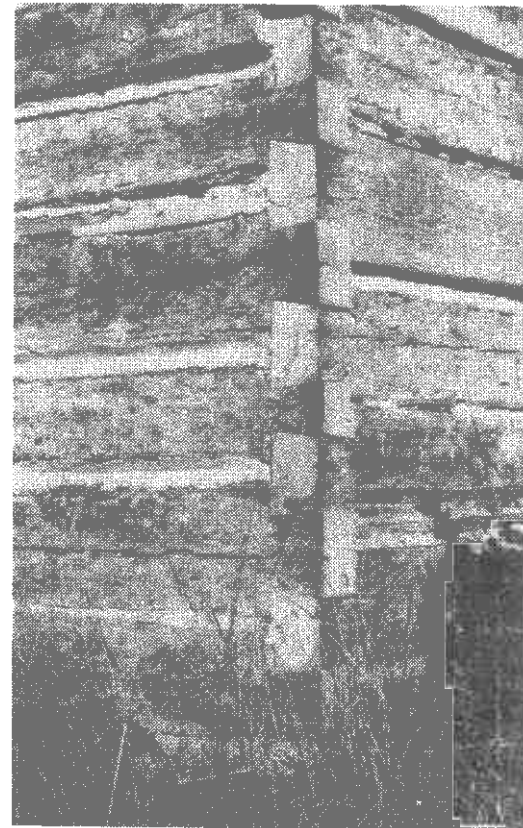
Detail of the dove-tailed corners in The McCoskrie Log House (1983 photo).
