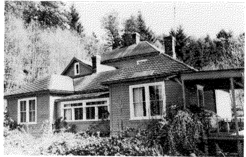
The Simson House, seaward side (1984 photo).
