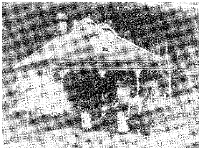
Original appearance of the front of the Ted Akerman House c. 1905 (courtesy Robert M. Akerman).
