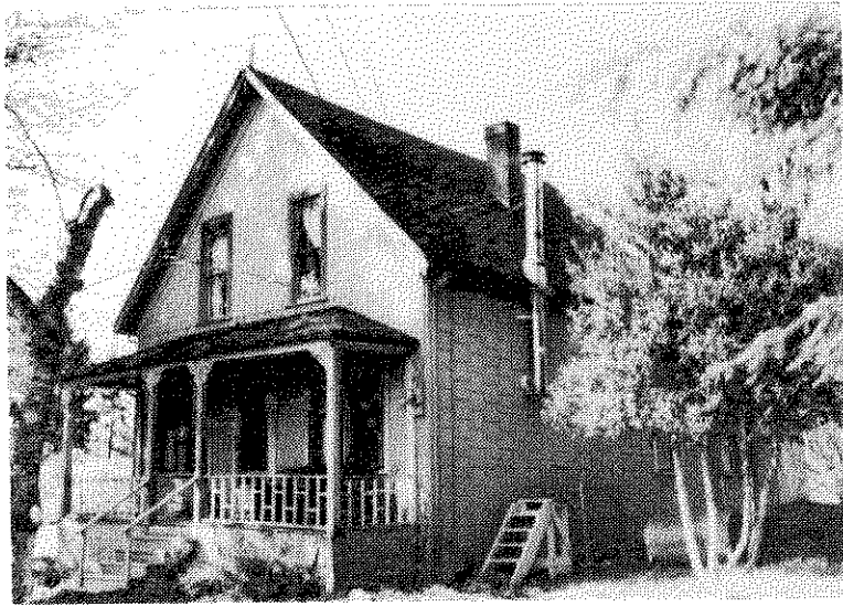
The Norton House (1984 photo).
