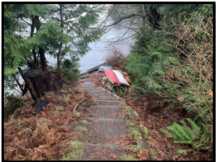
Photo 10. Stairs to the shoreline with boats left above high tide line.
