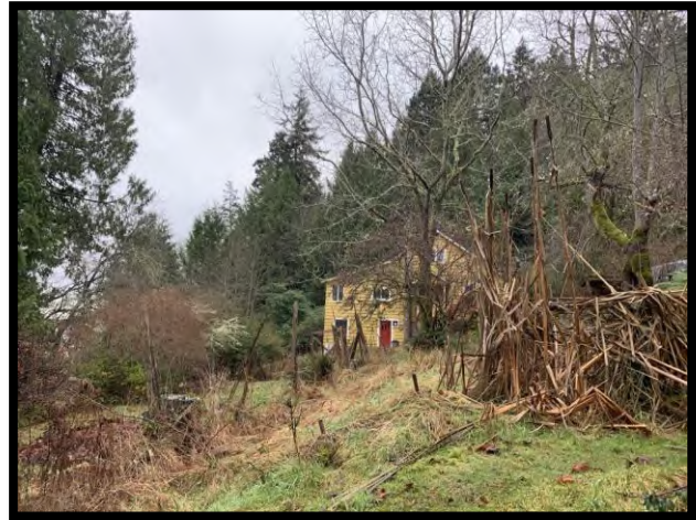
Photo 5. Vegetative tertiary filter wastewater treatment system on right and garden fence on left with house behind.
