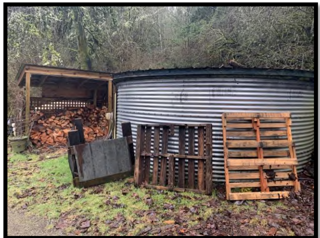
Photo 6. Water storage tank in foreground with woodshed in background next to house.
