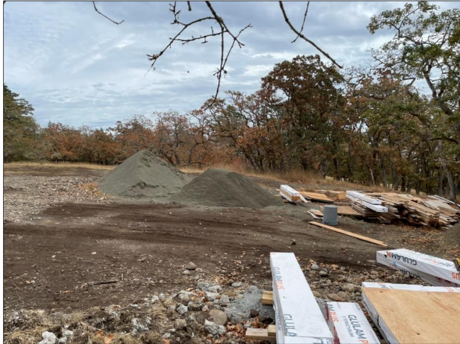
FIGURE 3. APPROX. LOCATION OF SEPTIC FIELD (RESTRICTIVE COVENANT J118502 AREA IN BACKGROUND)
