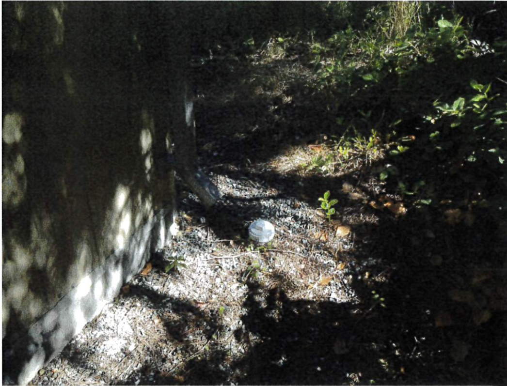
Photo 1. Downspout from roof, drains onto gravel pathway and infiltrates, in heavy rainfall runoff may flow through the vegetation to the right.
