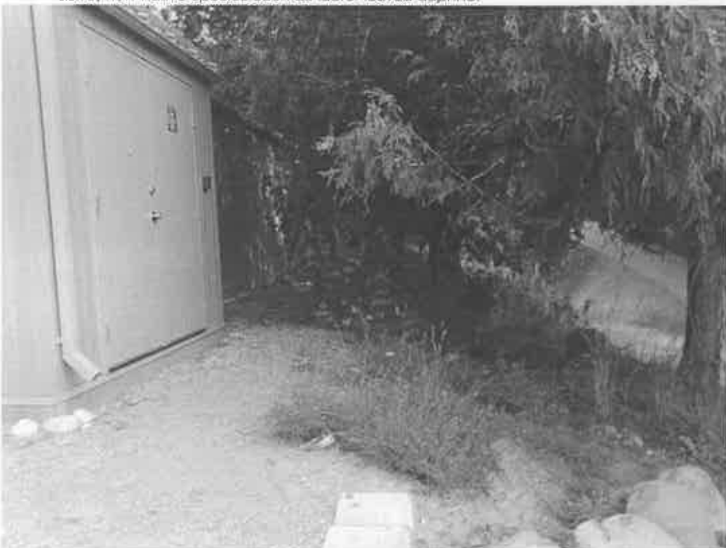
Photo. 4. Downspout from roof, drains onto gravel pathway and infiltrates, in heavy rainfall runoff may flow through the vegetation to the right.
