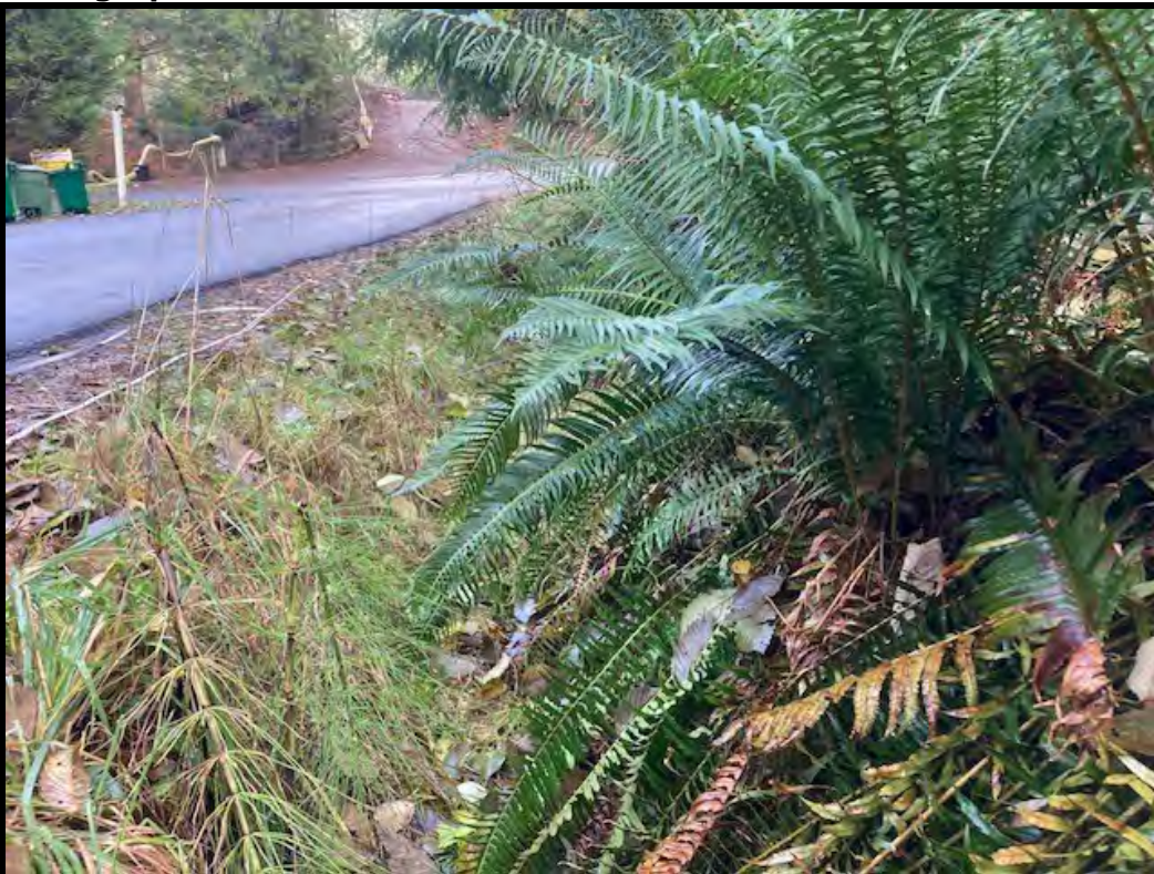
Photograph 14. View downstream Hikers Trail Road ditch.
