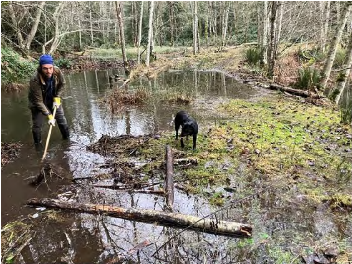
Photos 1 and 2: Flooding of the road through VLNR covered in water, January 7, 2025 due to beavers plugging the culvert located where the tool is being used to unplug.
