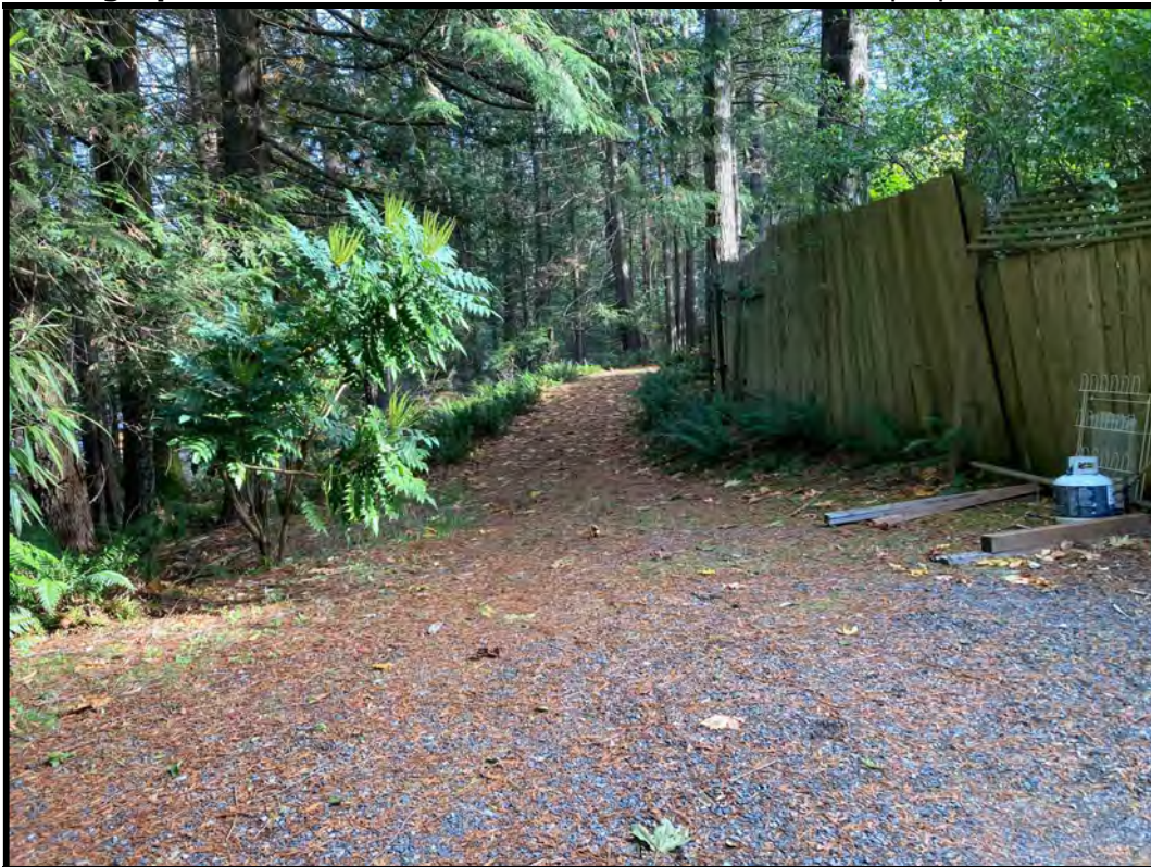
Photograph 2. View to the northeast of proposed access road to proposed cabins to be regraded.
