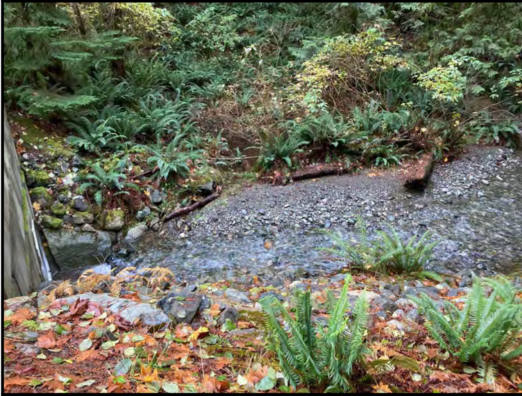
Photograph 13. View south of Kill Creek culvert inlet beneath Mount Gardner Road.
