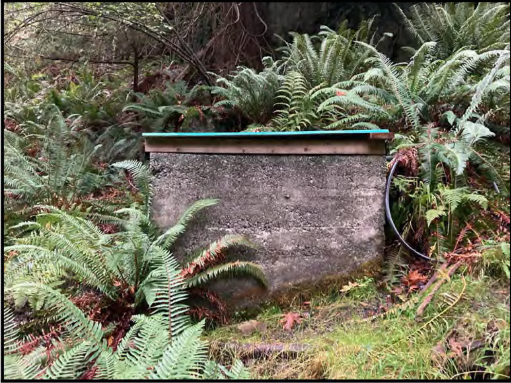
Photograph 5. 564 Collins Road, view to the northwest of existing well.
