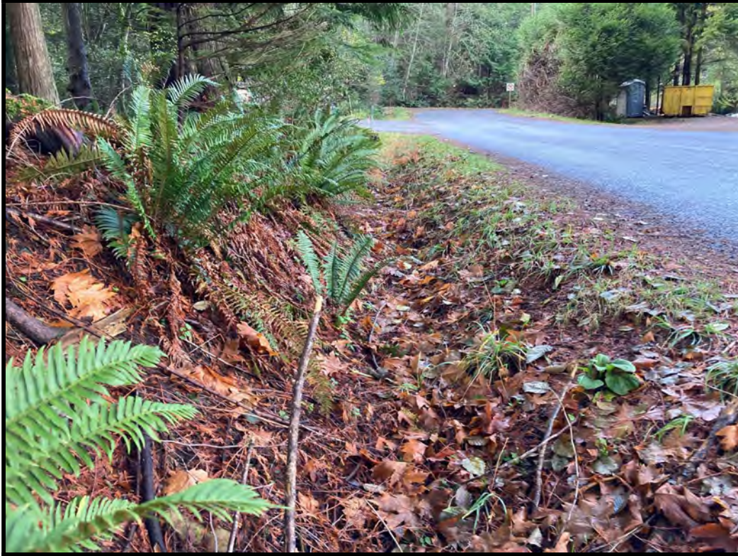
Photograph 15. View downstream Mount Gardner Road ditch.
