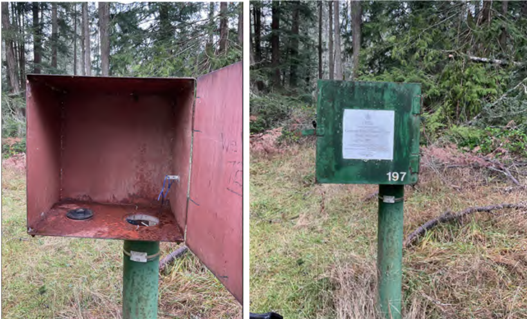
Figures 3 and 4: Current photos of Provincial Groundwater Observation Well Box 197.
