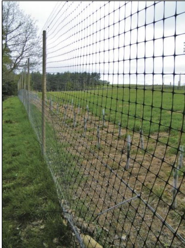
Figure 20: Example of temporary fencing
