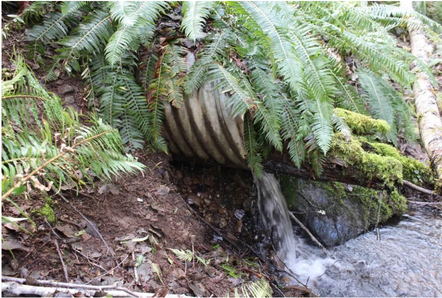
Photo 21. Culvert under trail at Boyle Creek. Culvert is perched and currently blocked with wood.
