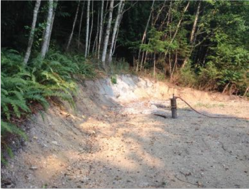
Figure 4 Area cleared for well head. Note colluvial deposits.
