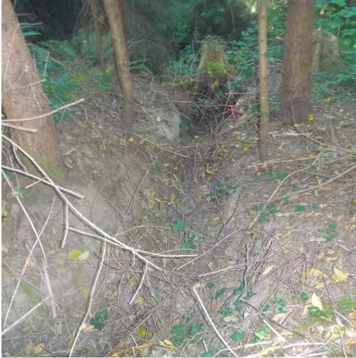
Photo 5: Erosion under stump and down ravine slope from pond outflow ditch
