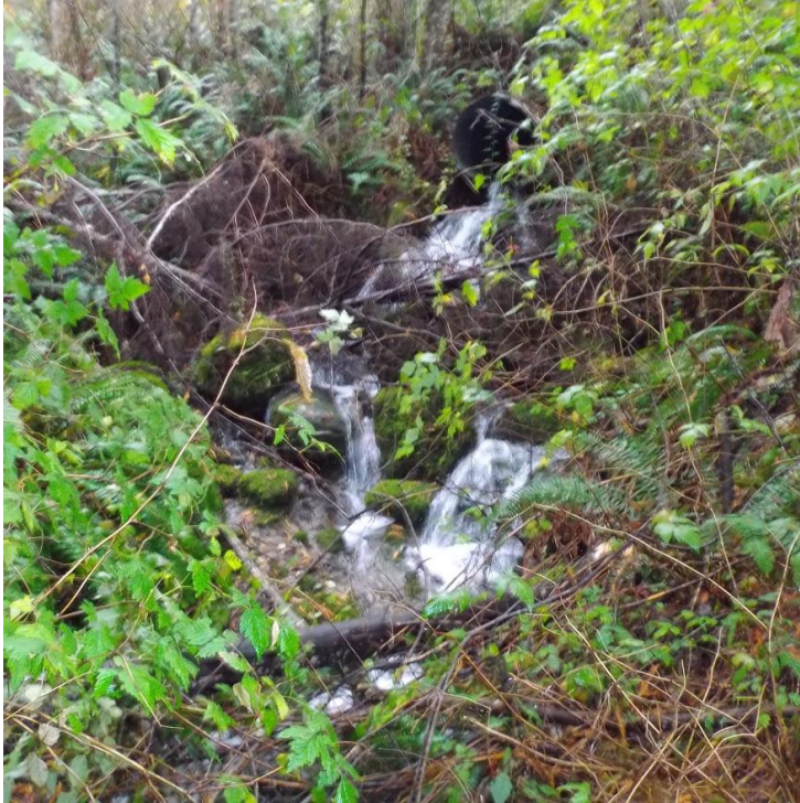
Photo 1: Ganges Creek outfall from driveway culvert near east boundary
