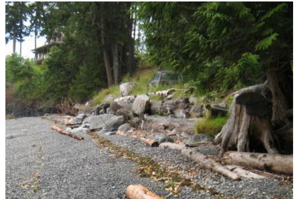
Wooden seawall and riprap boulders along shoreline – Lasqueti Island – Photo RC de Graaf
