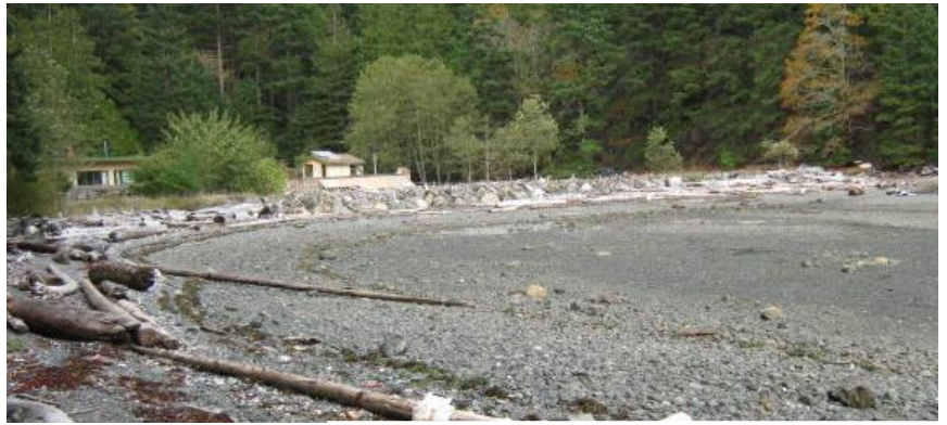
Seawall and riprap armoring on foreshore – Lasqueti Island Photo: RC de Graaf
