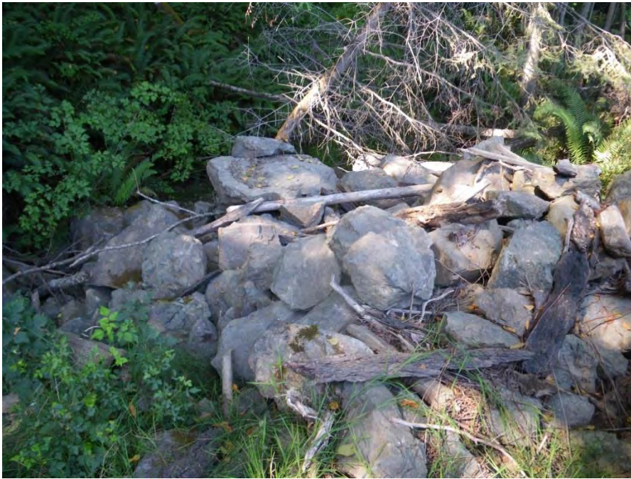
Photo 16. Looking downstream (west) from the outlets of the two culverts that drain Hadley Lake. During periods of high flow, water flows over the rip-rap boulders and into the defined channel at the base of the slope (marked with red arrow).
