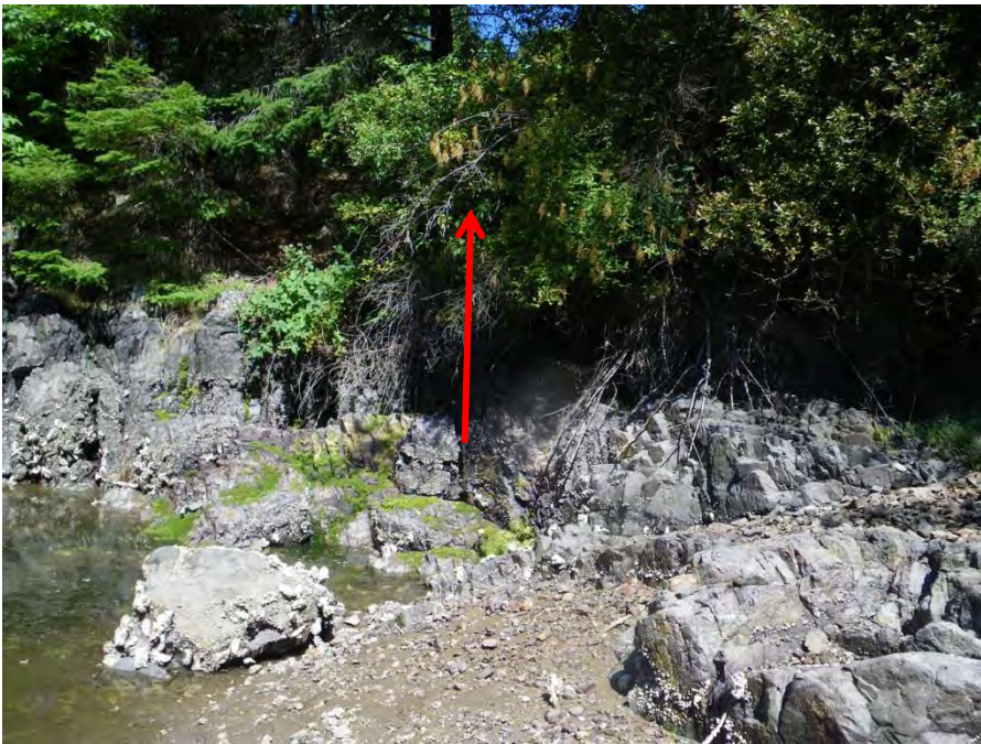
Photo 2. The outlet of Stonehouse Creek. Note the vertical bedrock ledge and lack of a plunge pool. Also, vegetation growth conceals the area where water flows over the ledge (marked with red arrow).
