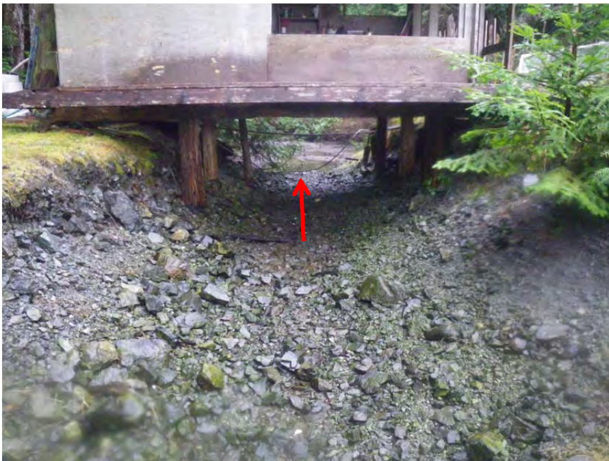
Photo 2. Looking upstream (south) at Mine Bay Creek from the natural boundary of the estuarine environment. Note the linear morphology of the channel, an indication that it was excavated. The red arrow indicates the point where the stream flows subsurface.
