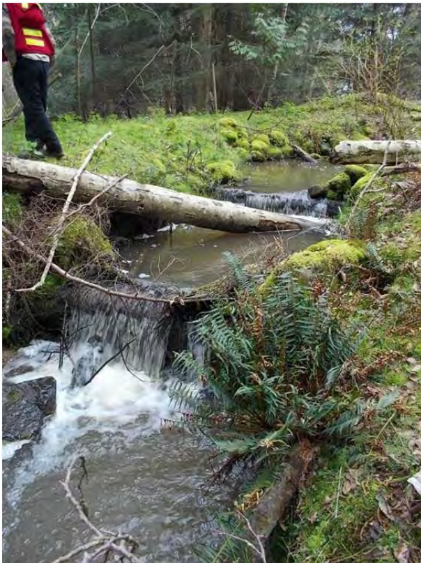
Figure 6. Photograph showing some of the in-stream features created to enhance fish habitat. Here, logs have been placed perpendicular to the stream and buried into each bank to create a cascade-pool channel habitat.
