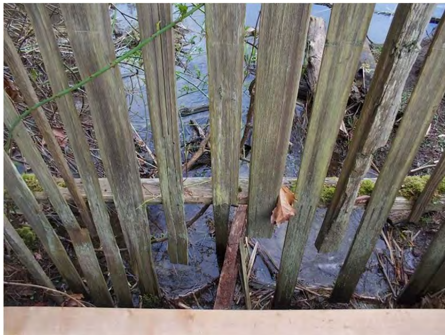
Figure 23. Looking down at the outlet from a bridge that crosses over the stream. Note that water flow from the pond is not impeded.
