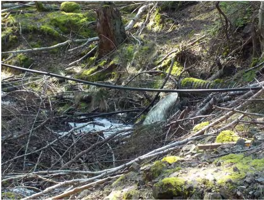
Figure 14. The outlet pipe from the dam, which drains the pond into the mainstem of the creek. This point is also the confluence of an Unnamed Tributary with Trematon Creek.
