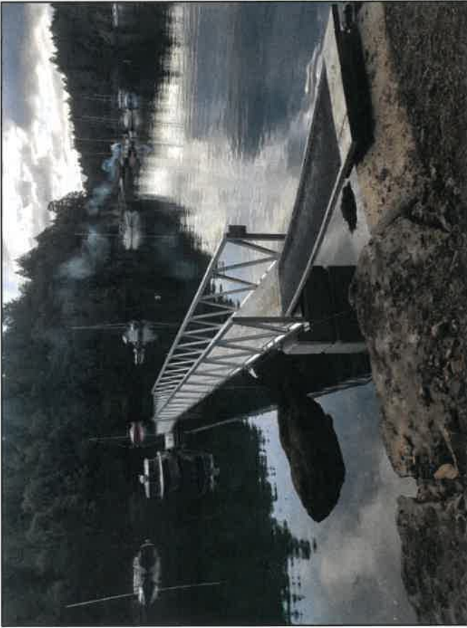
Photo10 & 11. Showing the new dock fronting Mr. Carey's parcel. The shoreline ramp and the end of the dock is supported on lock blocks. The second pier is on a natural bedrock with small wood piers. The third support is lock blocks. The dock is held in place by anchor chains to lock blocks.
