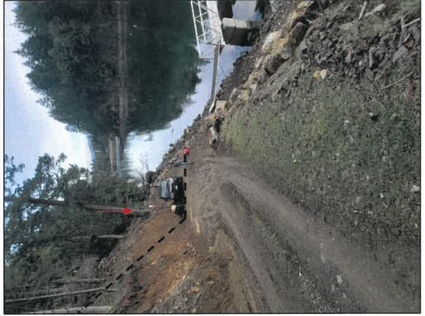
Photo 7-9. Showing the same section of shoreline post construction at a 3.6m tide looking across Mr. John Carey's shoreline and dock where the slope cut was further back into the slope to create the road. The property line (black dashed line) is approximately at the front of the pick-up truck.
