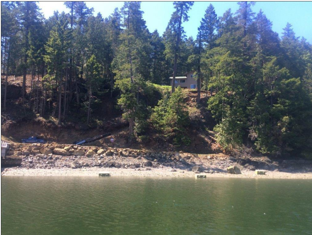
Figure 3. Photo of works (provided by FLNRORD staff).
