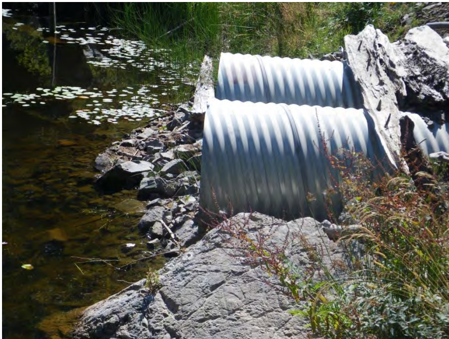
Photo 15. The inlets of the two outlet culverts that drain Hadley Lake. Note the summer-time water level of the lake is approximately 1.0 m below the bottom of the culverts.
