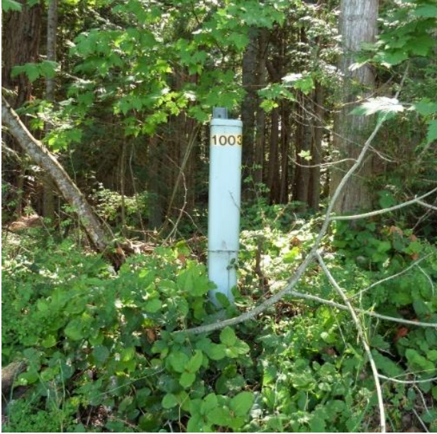
Photo 15. Old access housing for buried cable.
