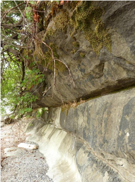
Photo 5. Cliffs along the northern shoreline.
