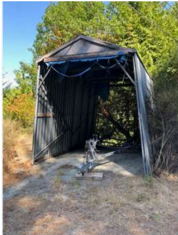
Front of shed
