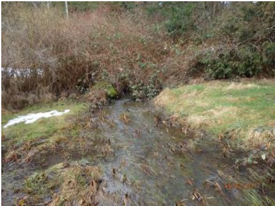
Characteristics of Reach 5 where the stream flows into the pond pictured above.
