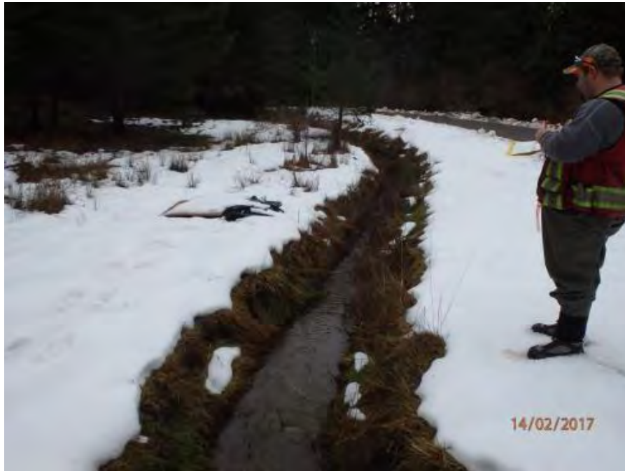
Looking downstream (north east) along the constructed ditch along the edge of Montrose Road close to the Mount Parke Regional Park parking area.
