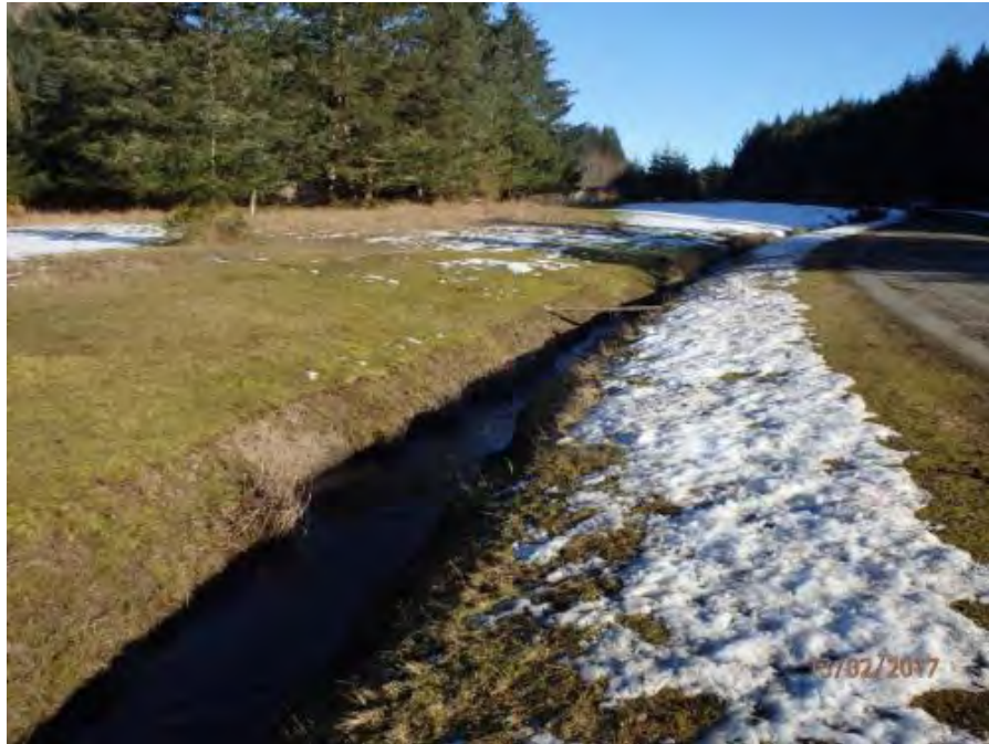
Looking upstream (east) along the ditch flowing along the north side of Merryman Road immediately upstream of its confluence with Deacon Creek.
