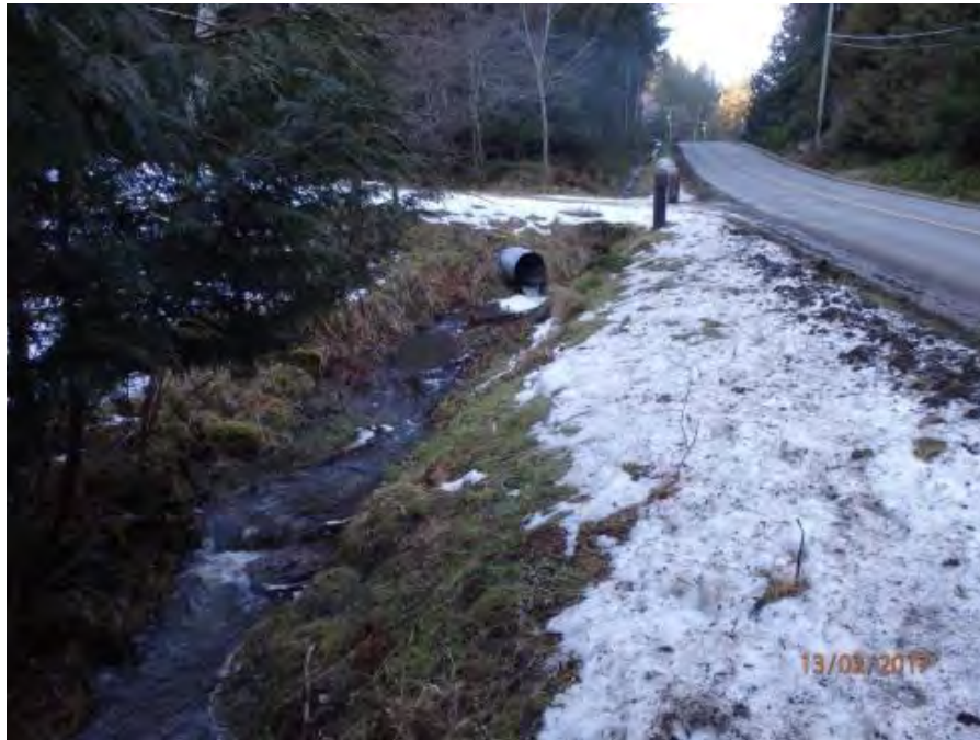
Looking upstream (north west) along the upper segment of Reach 2 where a culvert carries the flow underneath a property access driveway (523 Horton Bay Road).
