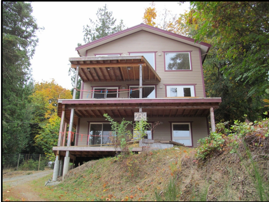
Photo 1 View of dwelling from Callaghan Crescent
