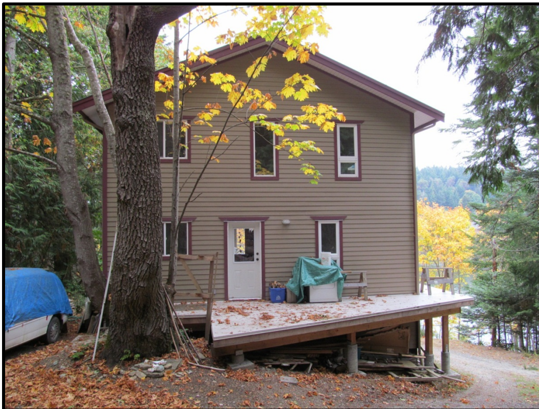
Photo 2 View of the rear of the dwelling showing large maple tree
