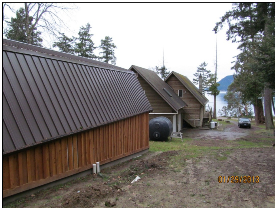
Picture 3: Looking west towards accessory building and Active Pass
