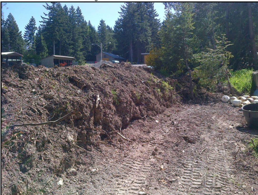
Figure 9: Berm being constructed between Highways Maintenance Yard and TUP site
