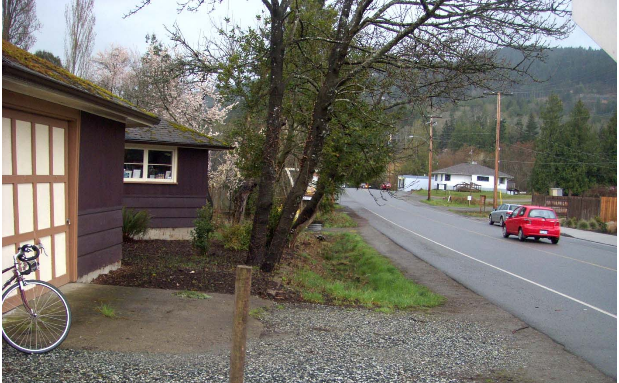
Figure 3: Looking south from north west corner of subject property, with parking space and drainage system viewed.
