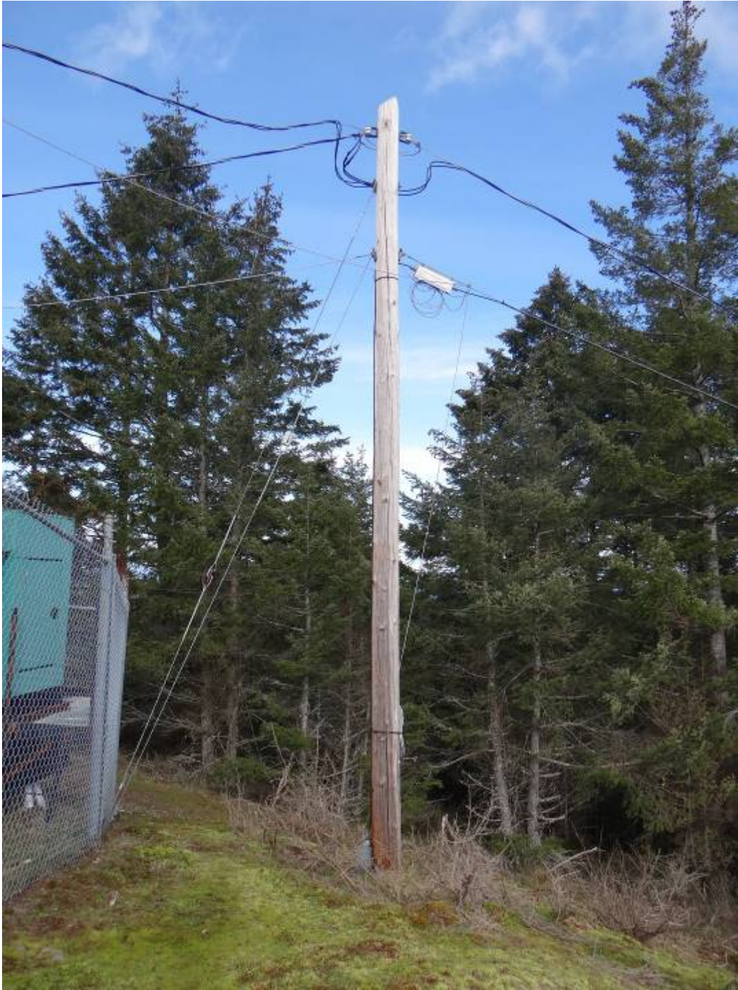
10. Hydro Service Pole – East of proposed compound
