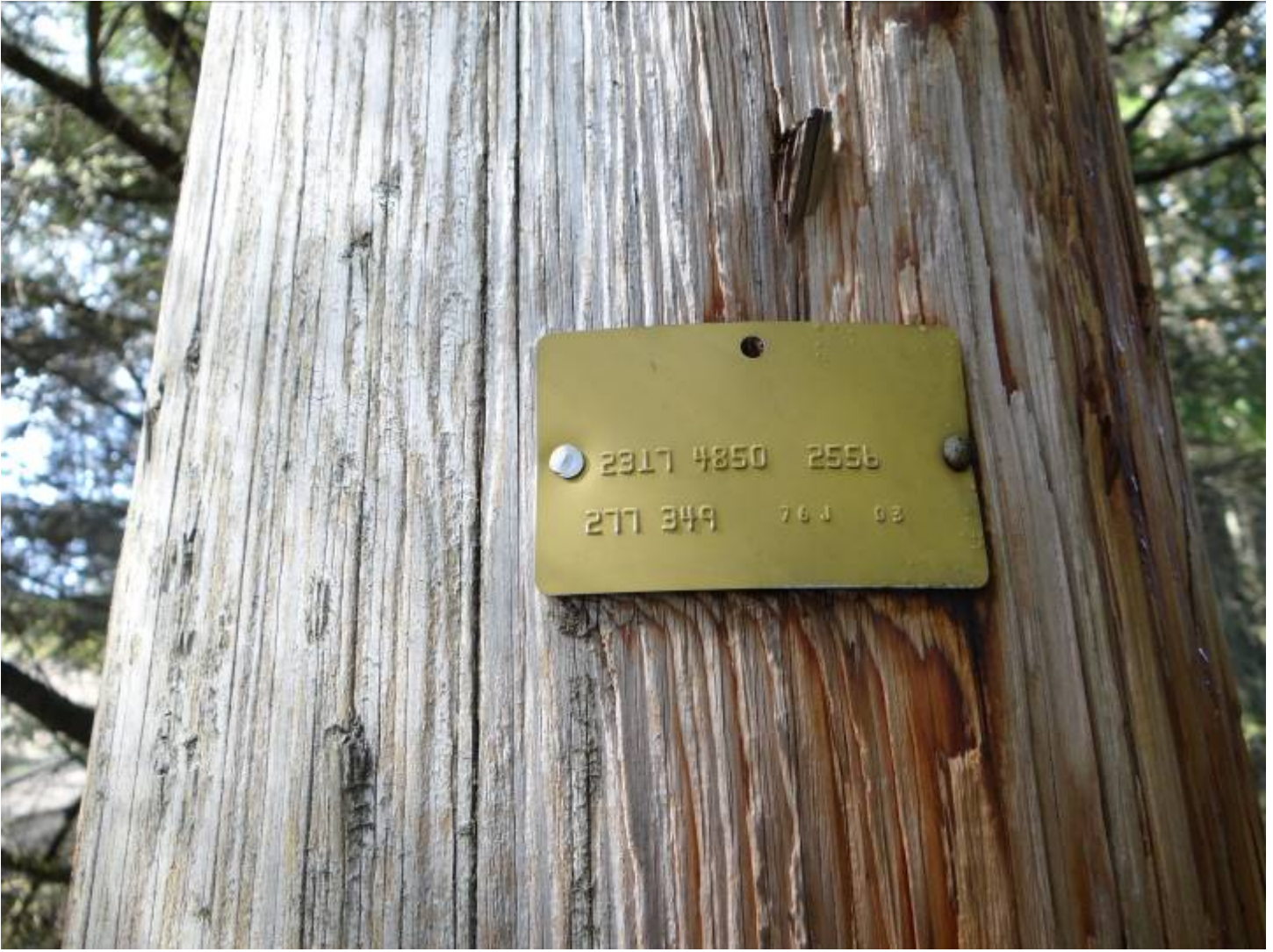
Hydro Distribution Pole Tag – South of proposed compound
