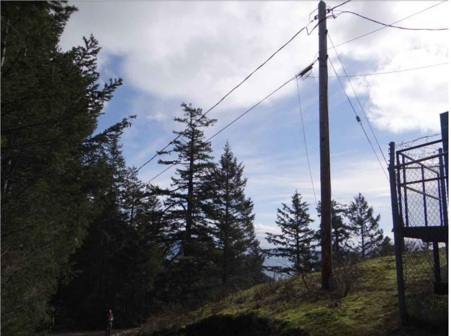
13. Guy Wire Easement Obstructions – Looking South West
