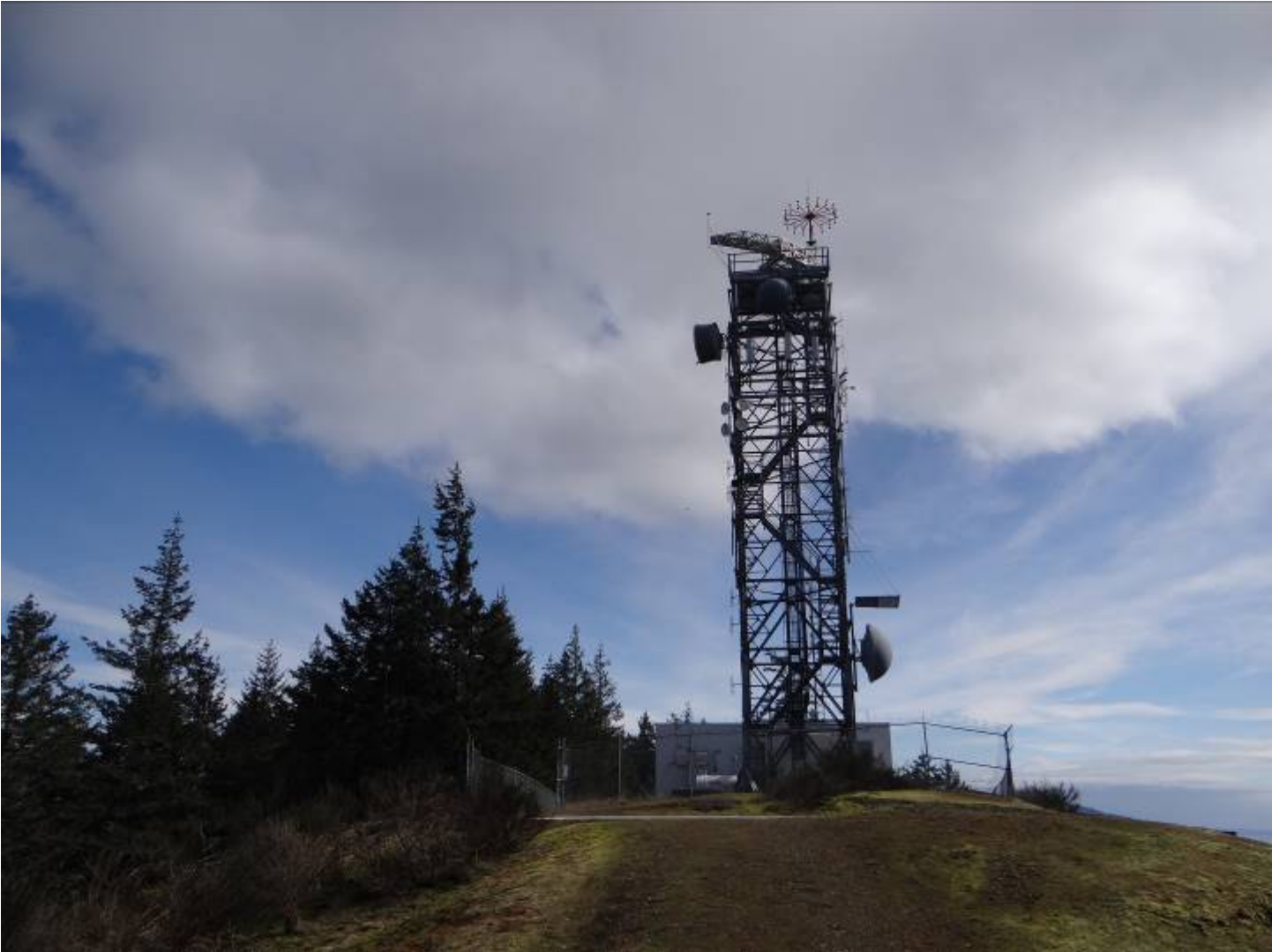
15. Existing Adjacent Tower – Coast Guard/Rogers
