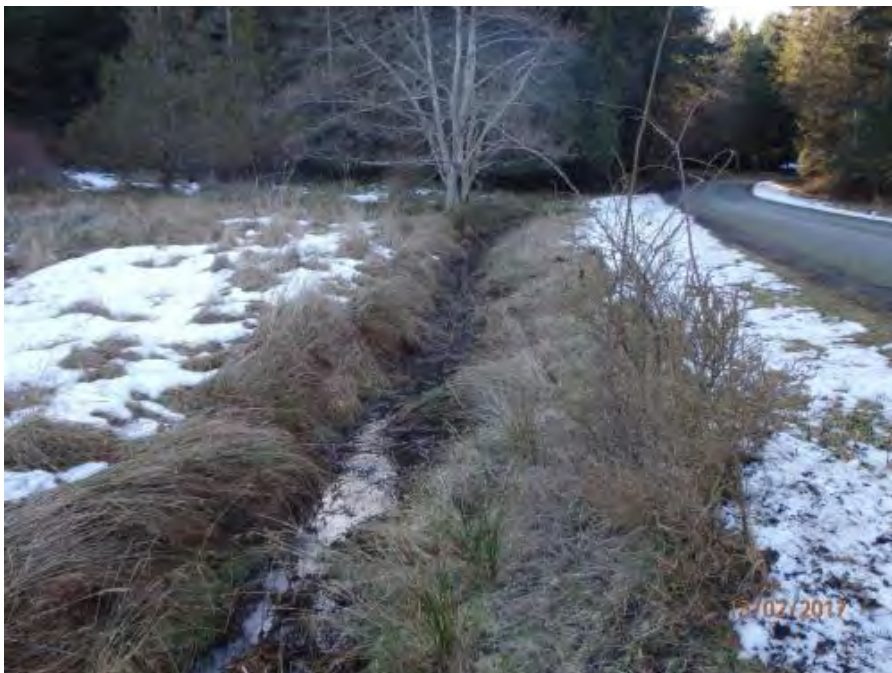
Looking upstream (west) along the ditch flowing along the south side of Merryman Road.
