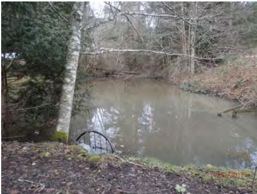
The dam shown above impounds water to form a small irrigation pond located mid-way through Reach 5.
