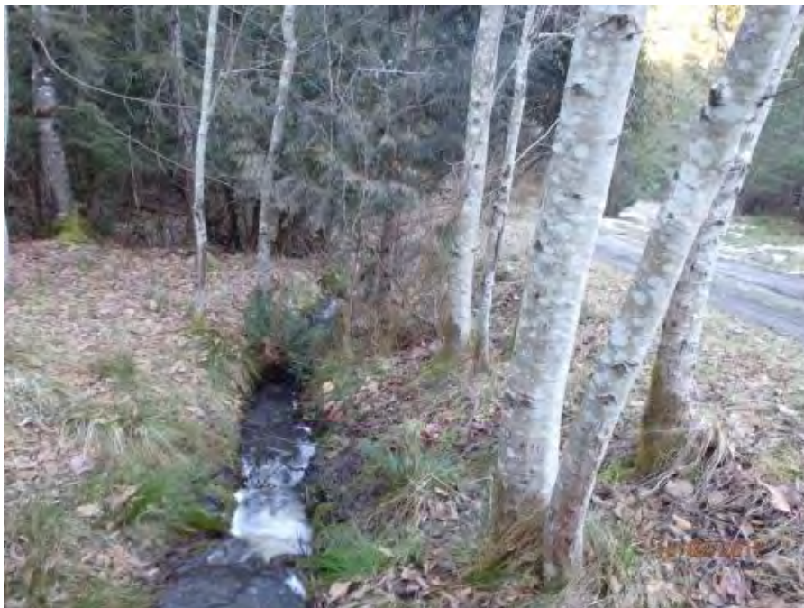
Upper segment of the ditch located on the 523 Horton Bay Road property.
