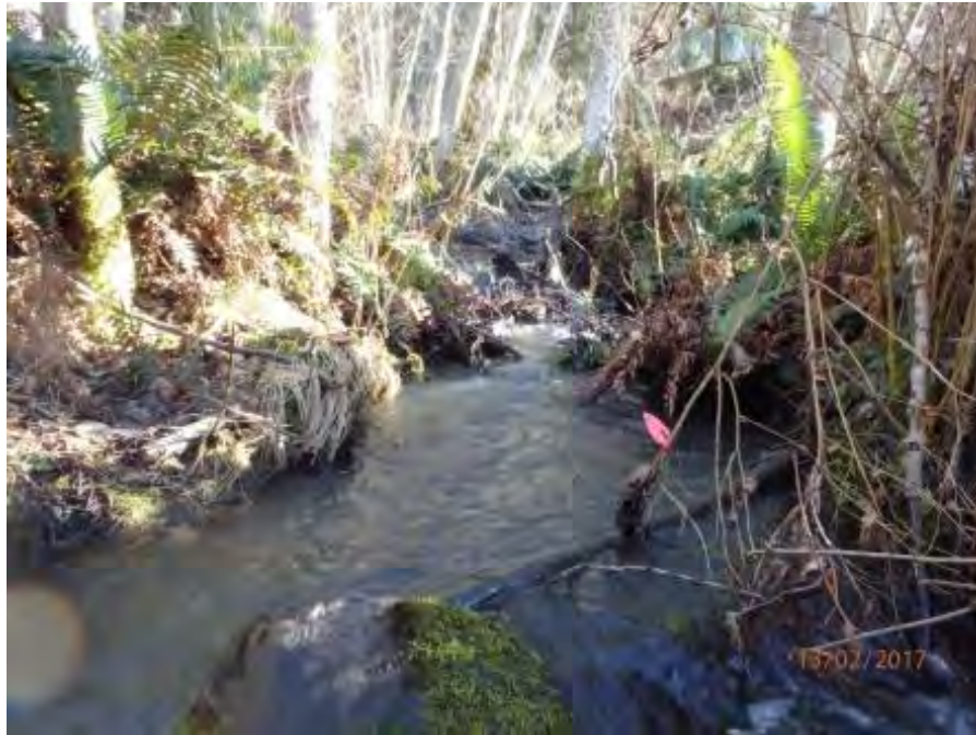
Looking upstream through the lower segment of Reach 2 from the Dalton Road culvert inlet. Note stable channel characteristics.
