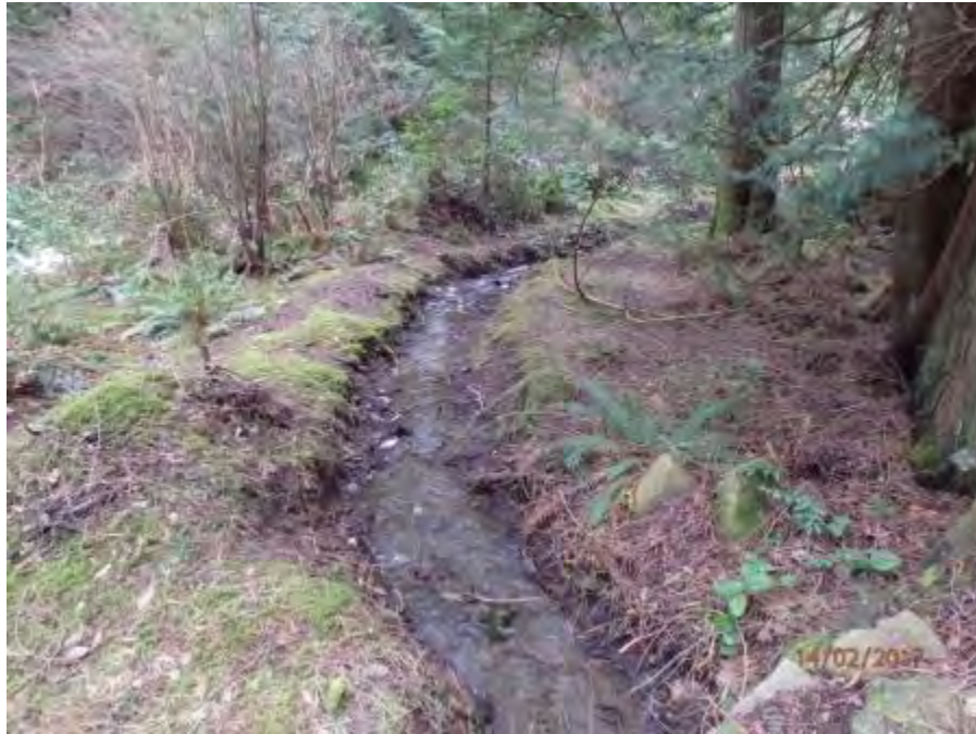
Looking downstream (east) along the ditch at the point where it flows out of the culvert under Montrose Road and onto private property.
