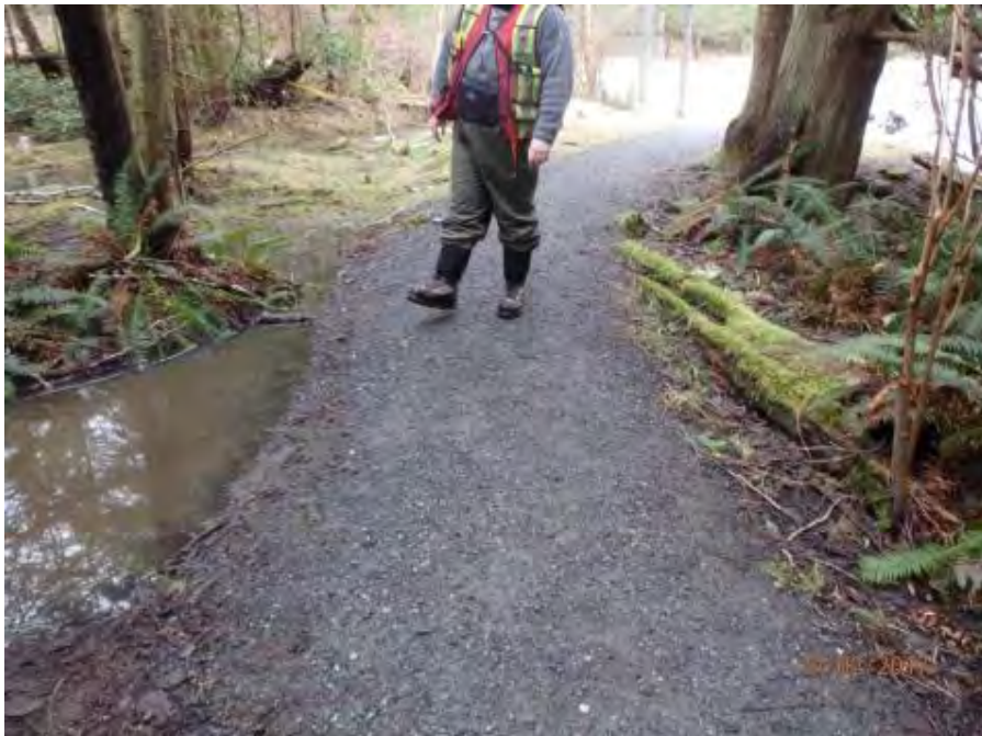
Foot trail to the immediate west of the photo shown above. Water is now directed via a constructed ditch along the north side of Montrose Road.
