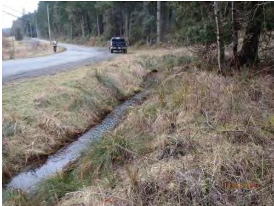
Looking downstream (south east) along Gallagher Bay Road close to the intersection with Horton Bay Road. The channelized stream flows underneath Gallagher Bay Road via two culverts at this location and represents the lower segment of Reach 2.
