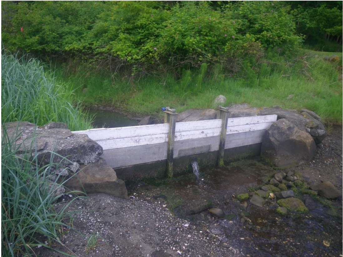
Weir that has been constructed where Deacon Creek flows out over the beach.
