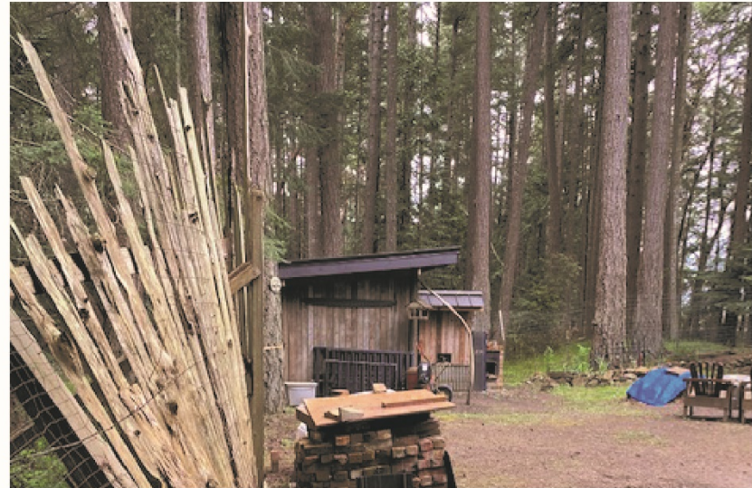
Recently constructed Woodshed and Water Storage Tank (southwest corner of property)
