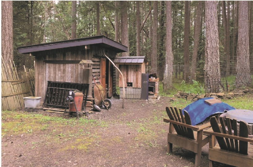
Recently constructed Woodshed and Water Storage Tank (southwest corner of property)
