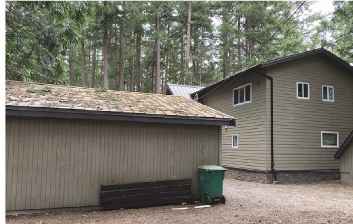
East side of Garage and Dwelling (view to west)
