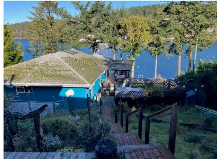
Dwelling (Looking to Miners Bay)
