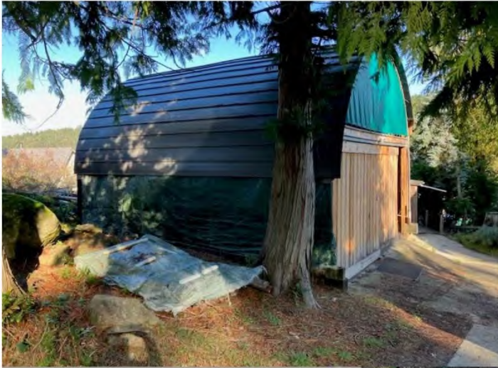
Front of Shelter from Road
