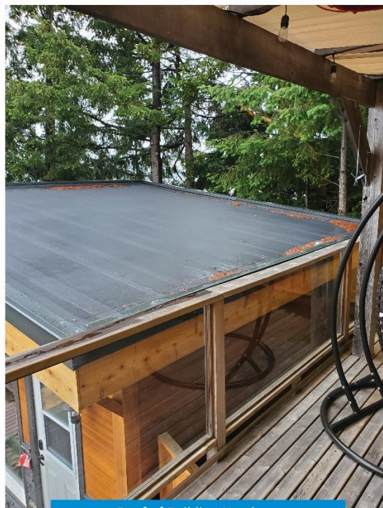
Roof of Building Northeast
