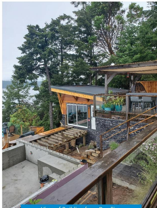
View of Building from Dwelling
