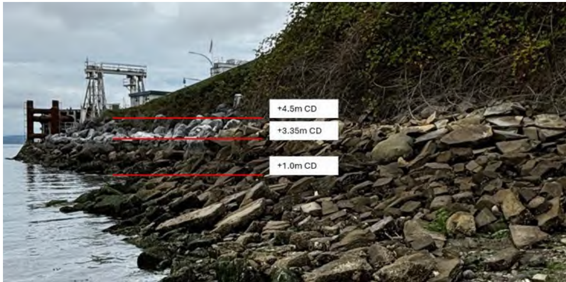
Figure 4-3 Zone 1 – Existing Riprap Elevations
