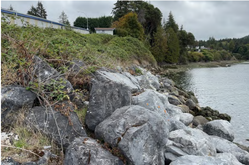
Figure 4-2 Zone 1 – Location A
