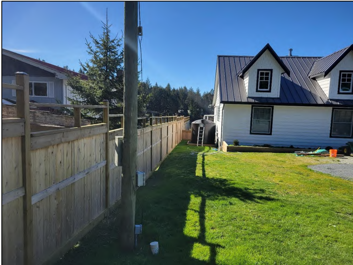
FENCELINE ADJACENT TO BUILDING SITE
