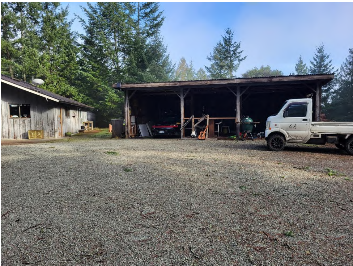
TEMPORARY KITCHEN BUILDING, LOOKING NORTH
