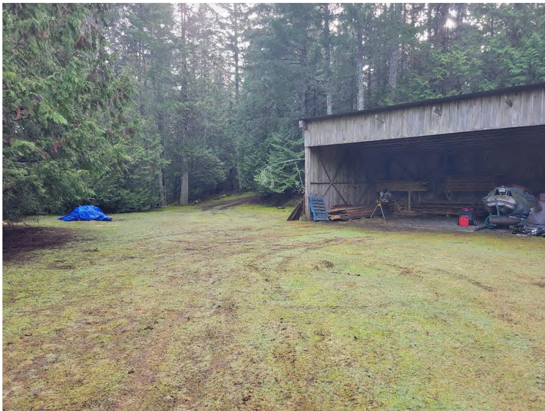
EXISTING HANGER BUILDING, LOOKING SOUTH-EAST
