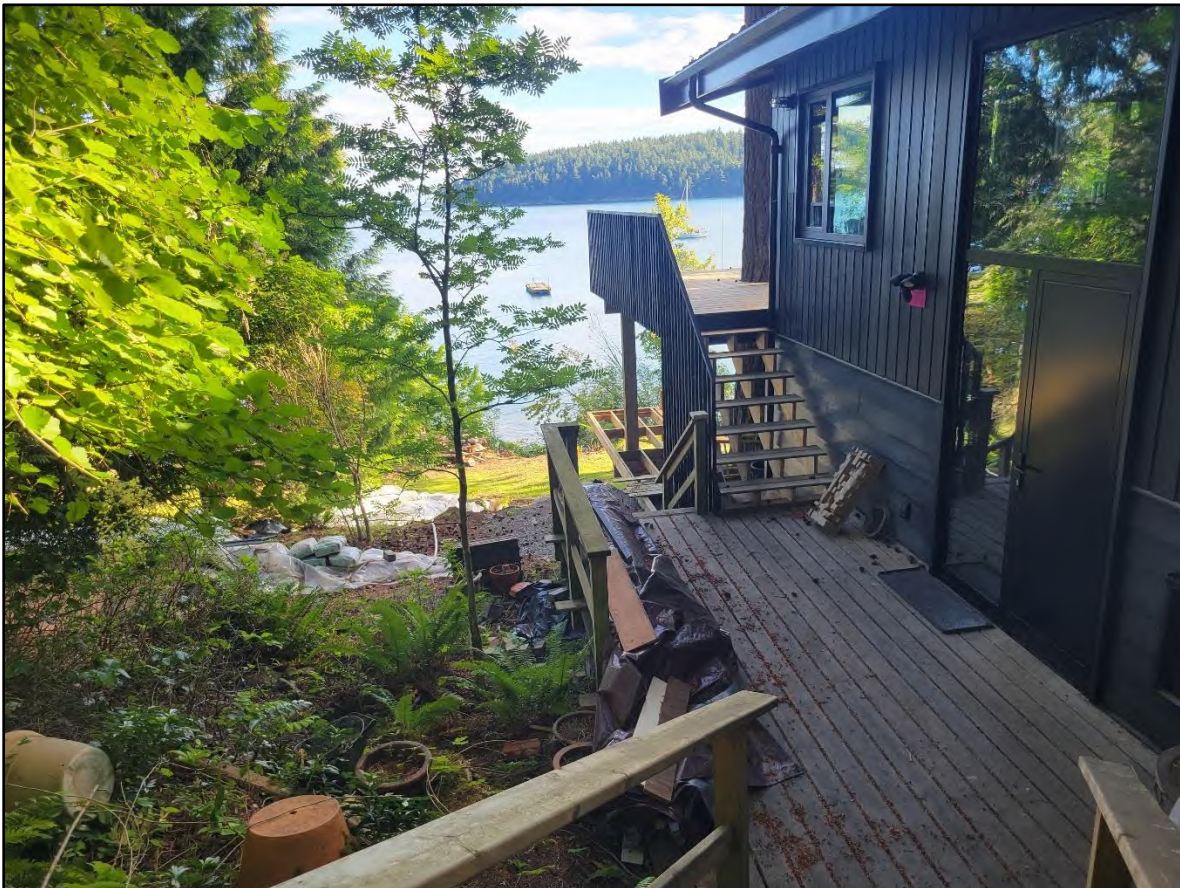
ENTRY DECK, LOOKING NORTH ALONG PROPERTY LINE
