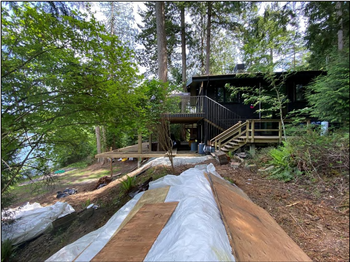
NEW DECK AND ENTRY STAIRS, LOOKING EAST
