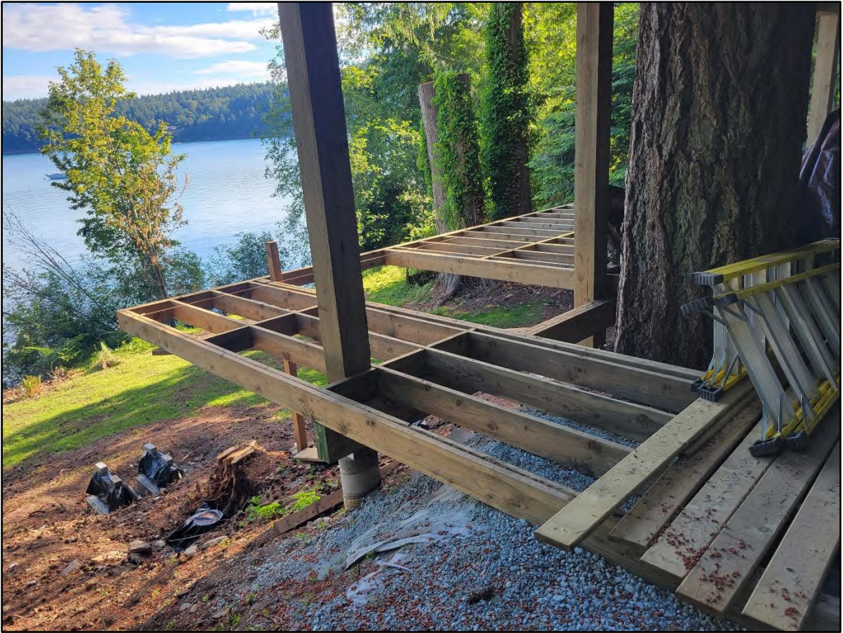
LOWER DECK AND FORESHORE ACCESS STAIRS FOUNDATION, LOOKING NORTH-EAST
