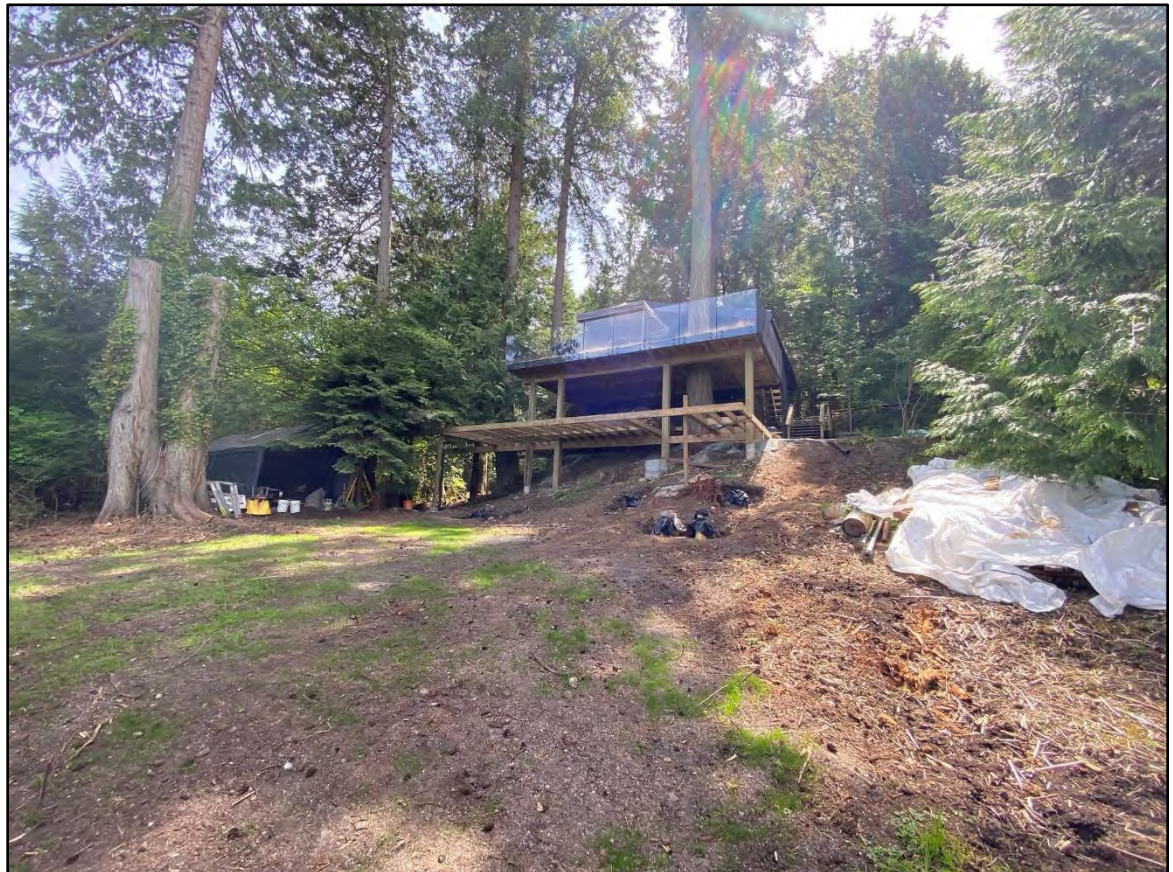
NEW DECK AND ENTRY STAIRS, LOOKING SOUTH
