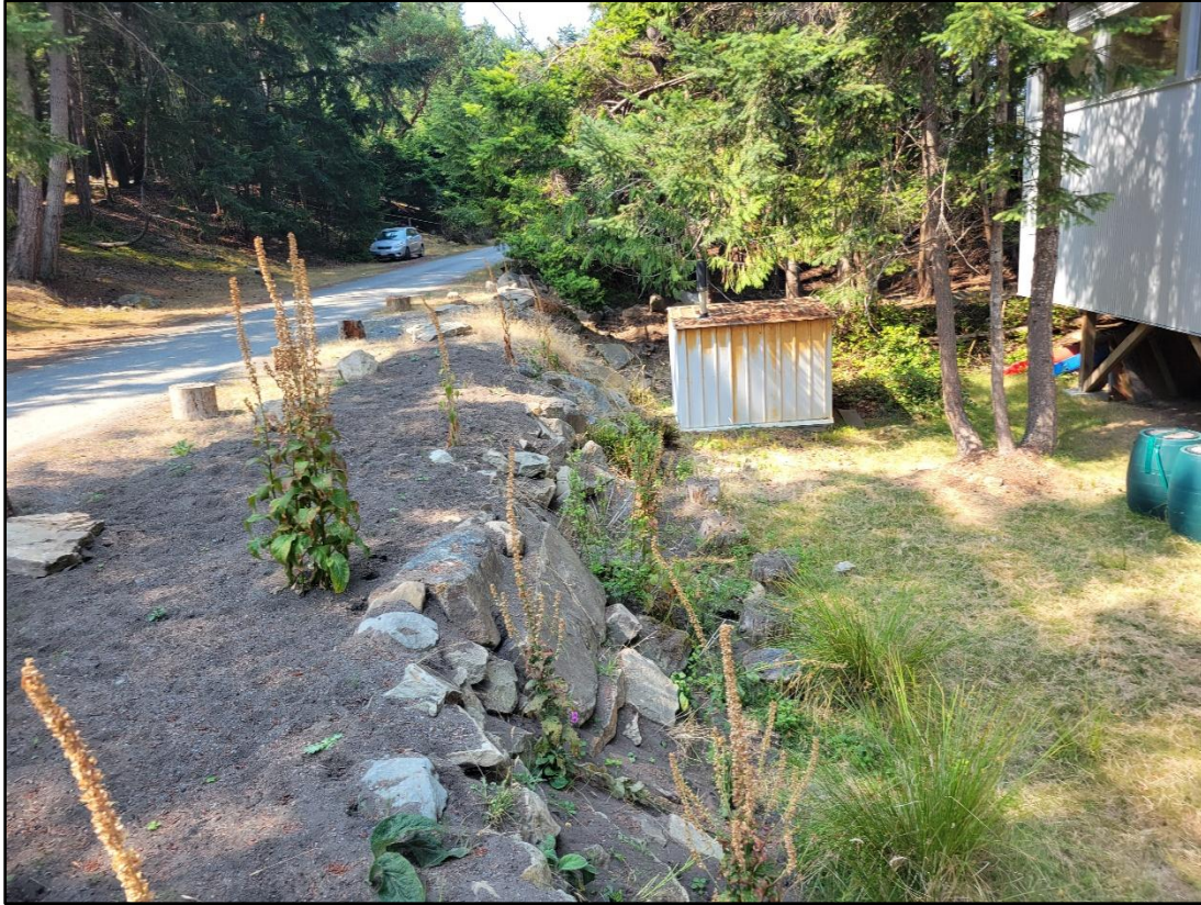
EXISTING RIP-RAP/ ROAD RETAINING WALL, LOOKING WEST
