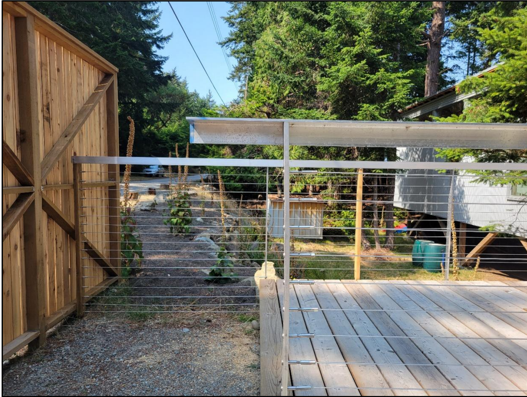
EDGE OF DECK ENTRANCE STRUCTURE, LOOKING WEST
