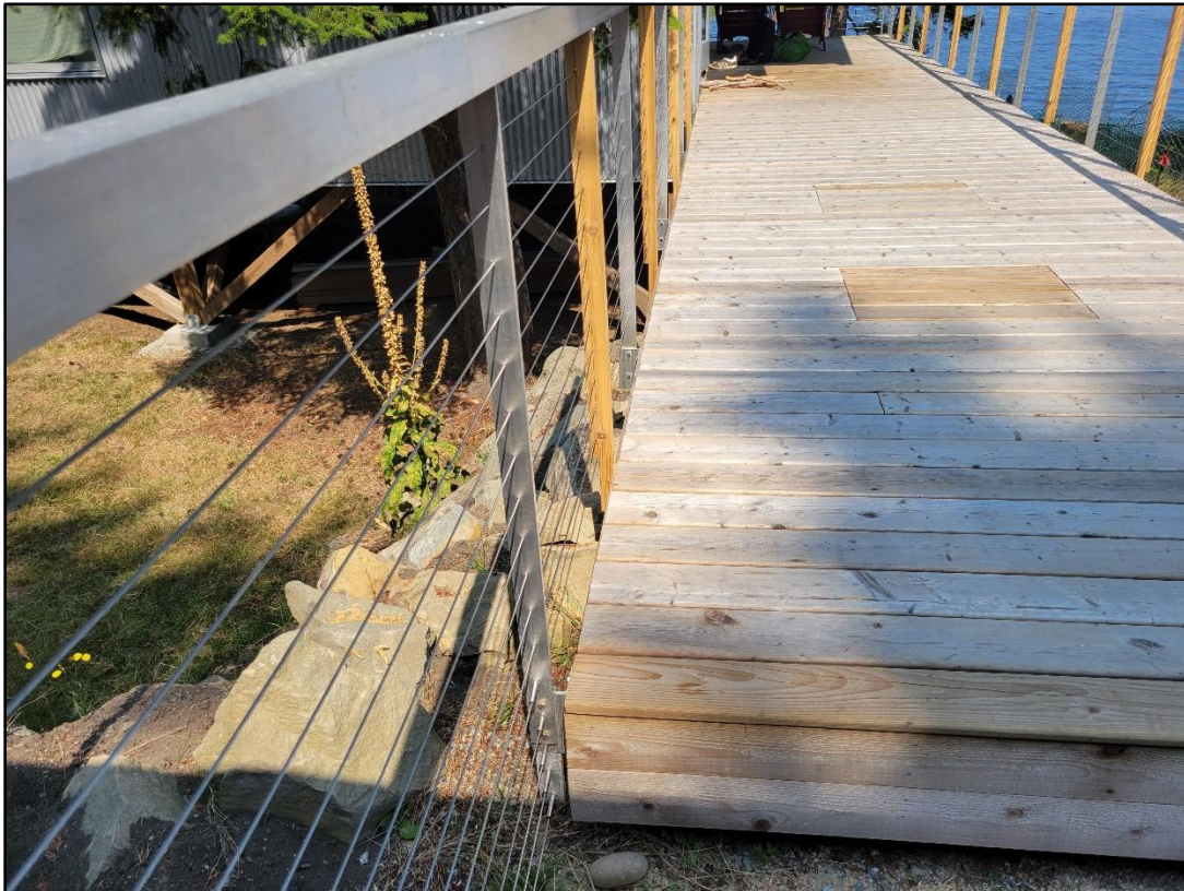
EDGE OF DECK ENTRANCE STRUCTURE, LOOKING NORTH
