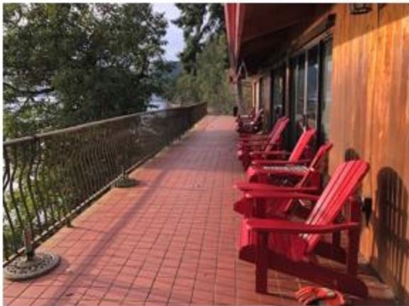
View of Deck
