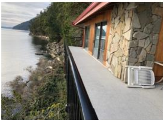
North East corner of deck (long view)
