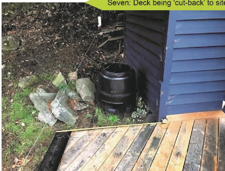
Seven: Deck being 'cut-back' to site entirely on property
