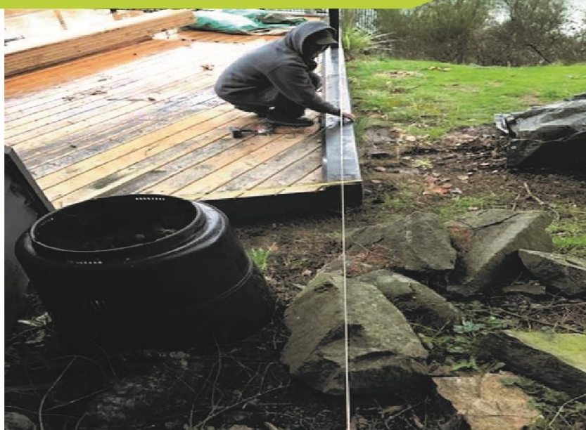
Eight: Deck being 'cut-back' to site entirely on property
