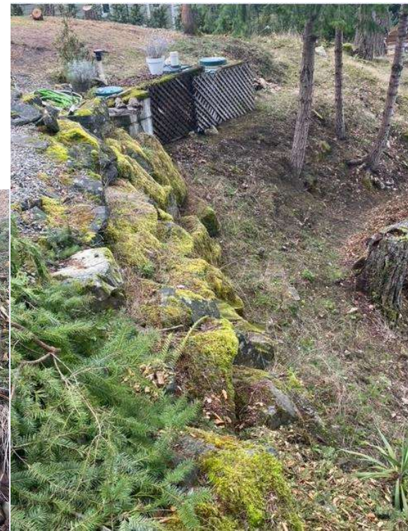
Photo 4. Side View of Retaining Wall
