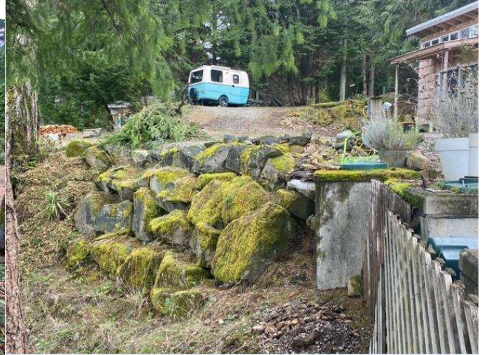
Photo 2. Existing retaining wall
