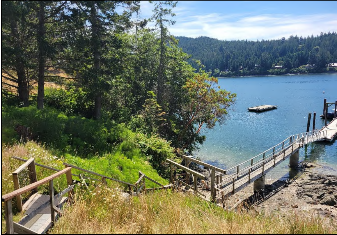
EXISTING STAIRS, DOCK, AND BOATHOUSE FOUNDATION, LOOKING SOUTH-EAST
