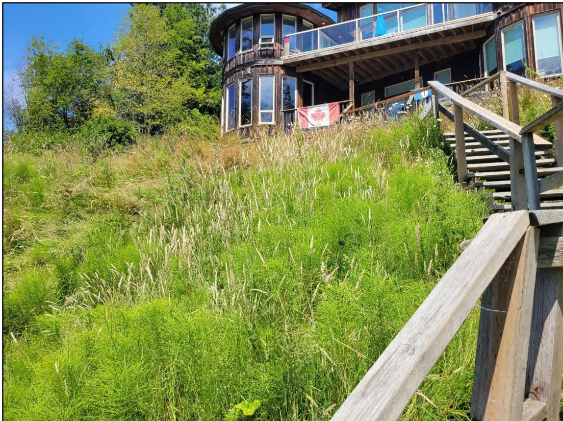
EXISTING STAIRS, LOOKING NORTH UP SLOPE TOWARDS EXISTING DWELLING
