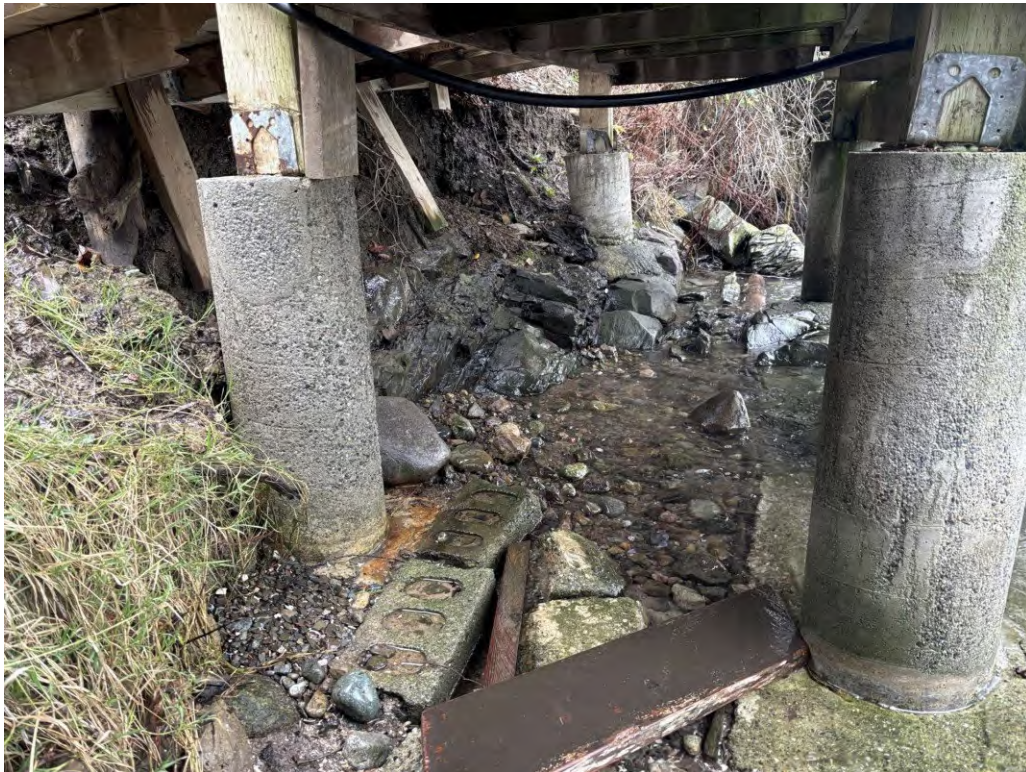
Photograph 3: Remnant concrete foundations from the boathouse.
