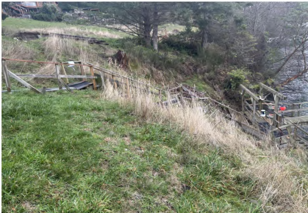
Photograph 2: View of slope and staircase, looking east.
