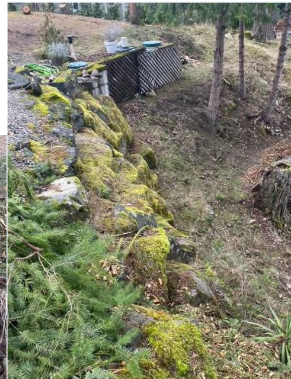
Photo 4. Side View of Retaining Wall
