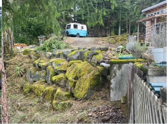
Photo 2. Existing retaining wall
