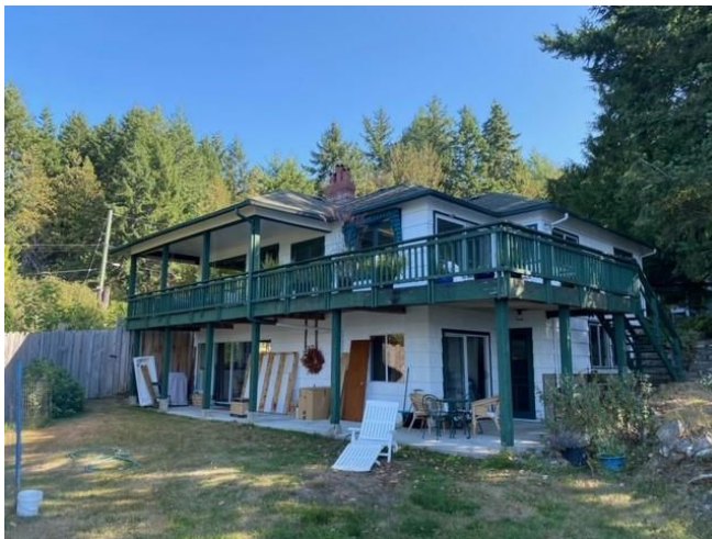
Photo 1. Broad view of back of House
