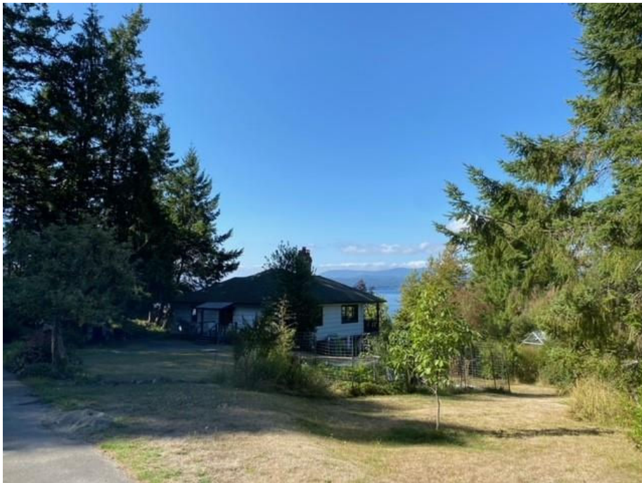
Photo 5. House from Road
