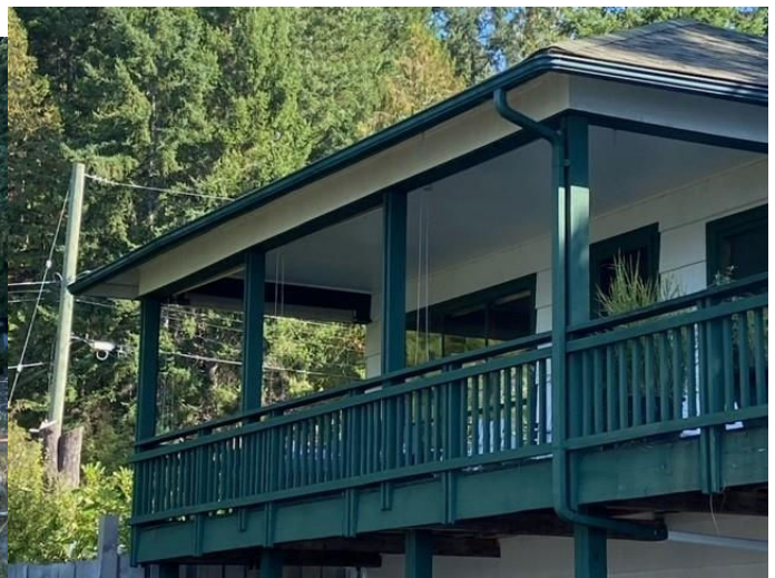
Photo 2. Corner of Existing Deck to be Closed-in
