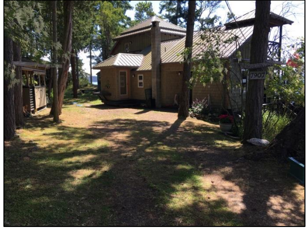
Image 10: Area of proposed dwelling unit addition, looking east. Note existing woodshed in left of frame.
