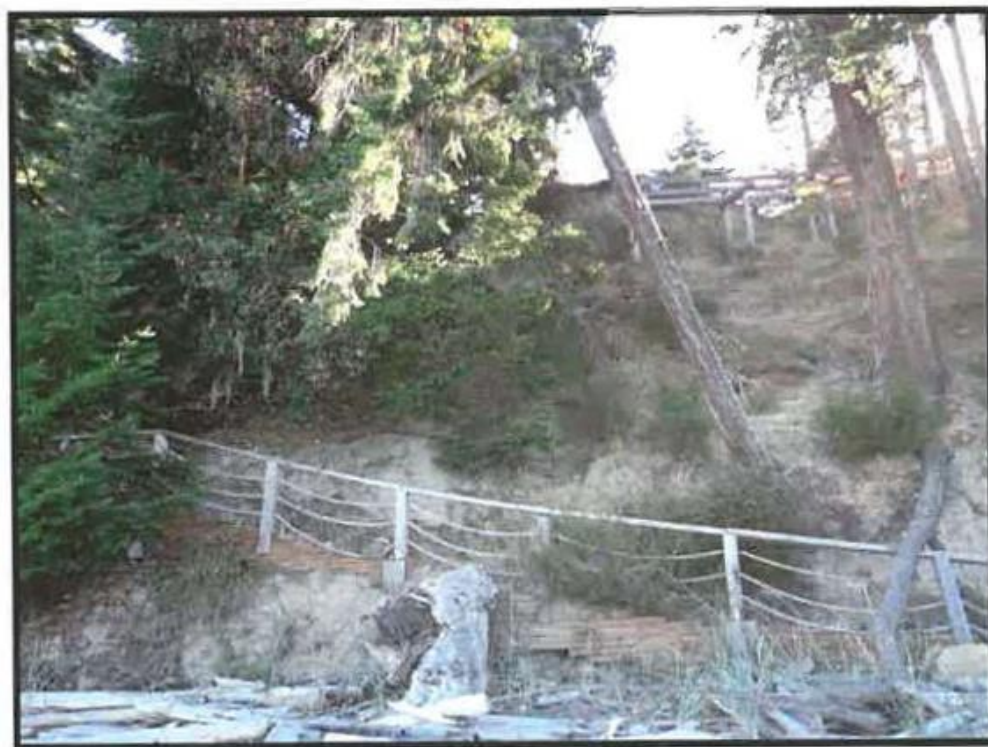
Plate 2: Looking upslope from the beach at remnants of old structure
