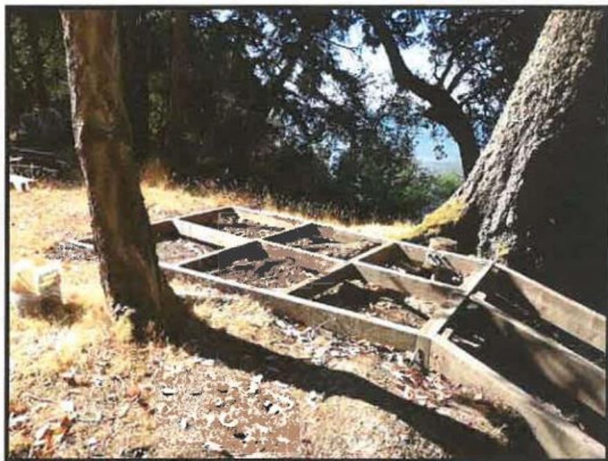
Plate 8: Platform for access structure at top of slope
