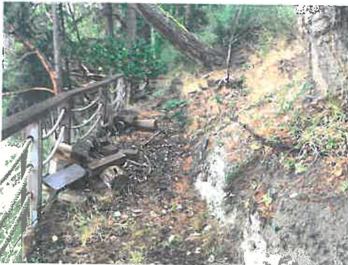
Below: Soil cut pathway with wood retaining wall along left edge, looking north
