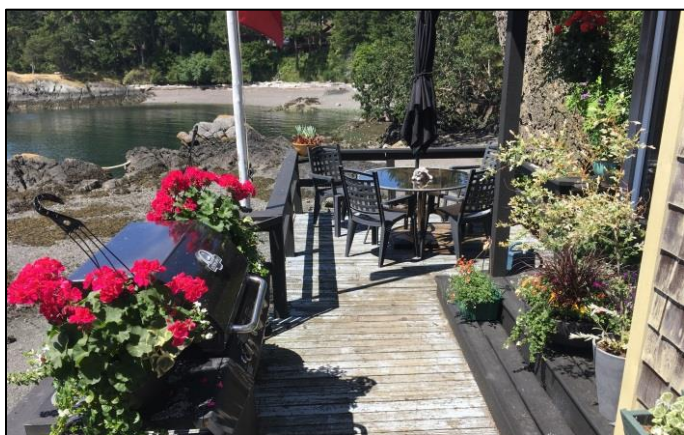
Image 3: Existing old deck, looking southwest
