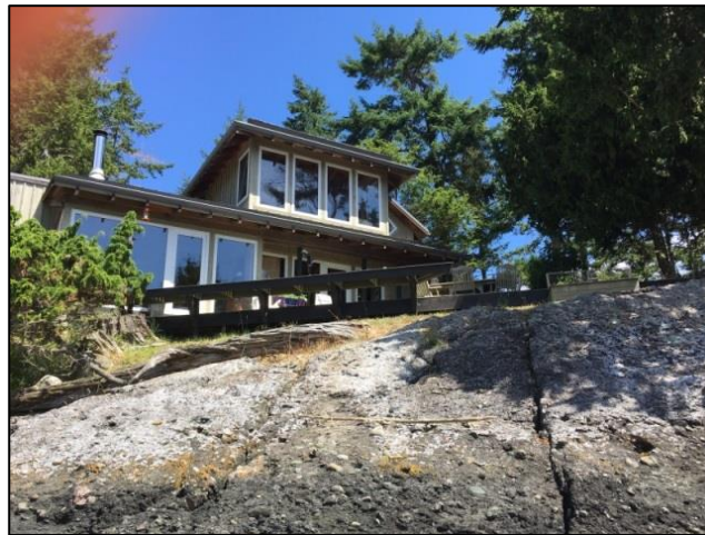
Image 8: Existing new deck, viewed from natural boundary of the sea.
