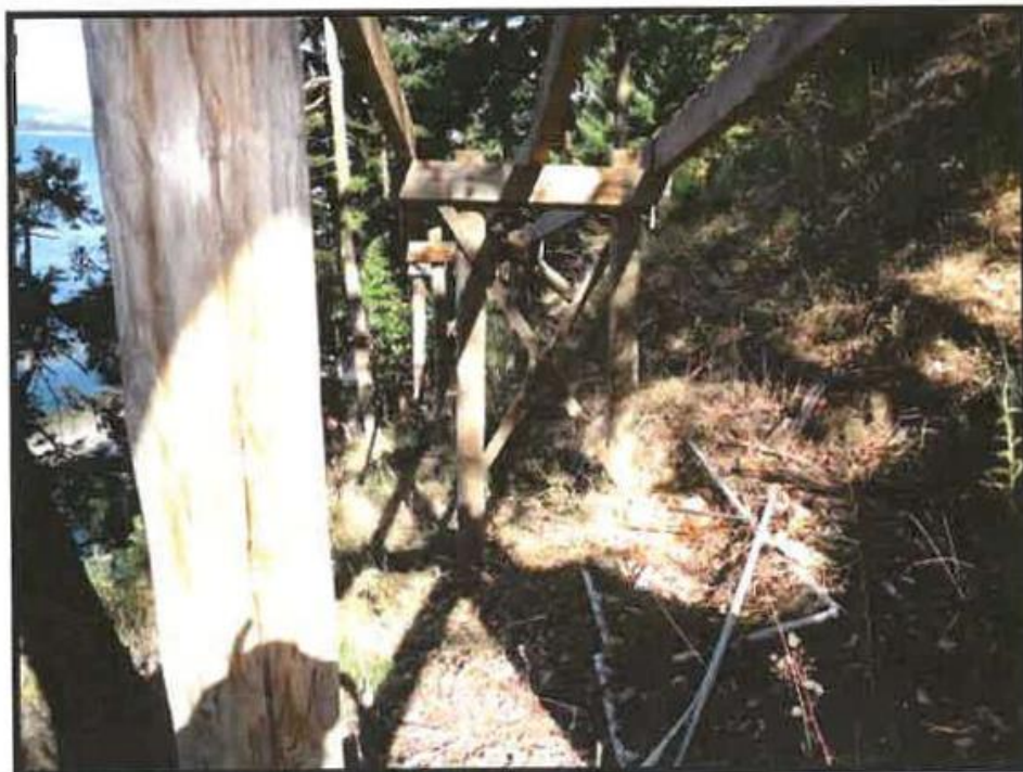
Plate 6: Looking downslope along the frame of the upper part of the access structure
