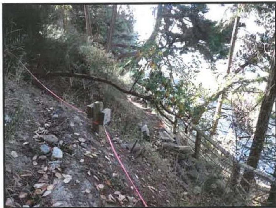
Plate 5: Looking south along the slope along the original alignment of access structure
