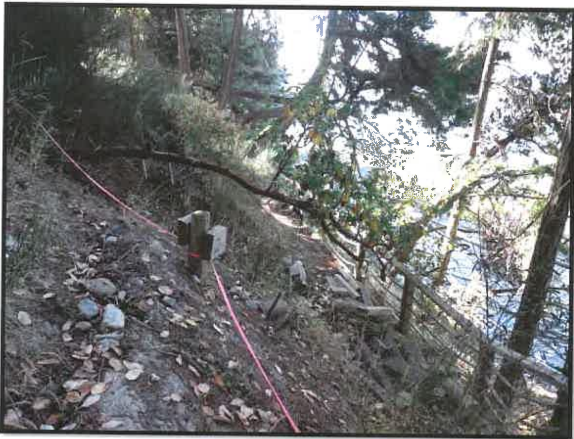
Plate 5: Looking south along the slope along the original alignment of access structure
