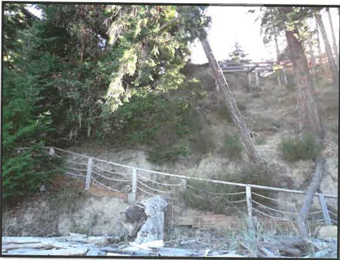
Plate 2: Looking upslope from the beach at remnants of old structure
