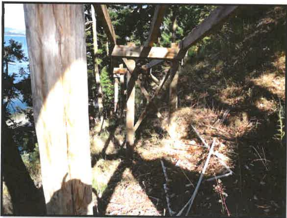
Plate 6: Looking downslope along the frame of the upper part of the access structure
