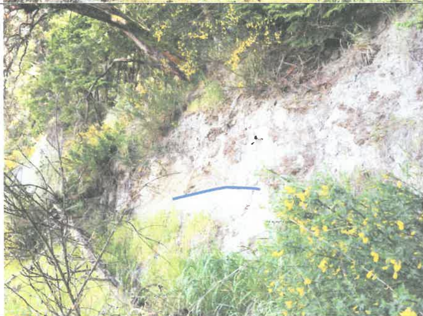
A soil scarp near top-of-slope on Lot 81, showing till (darker) over sand. The blue line is along the division between the soil types.
